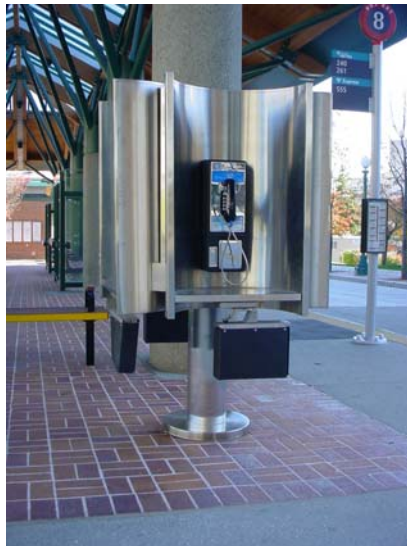
Figure VIII-5 Example of Shelter/Telephone Installation at Bellevue Transit Center
