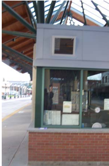
Figure VIII-10 Bellevue Transit Center Real-Time Monitor (above information booth)
