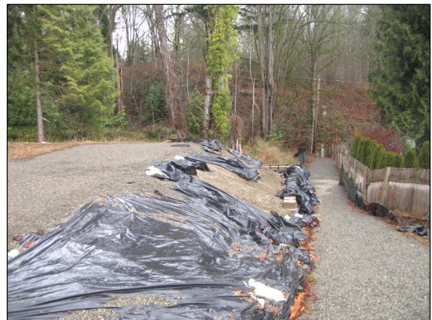
Looking north from position 2 – New Trail
