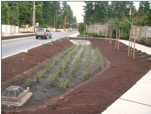
Rain Garden on the west side of 145 th PI SE north of 144 th Ave SE, looking south
