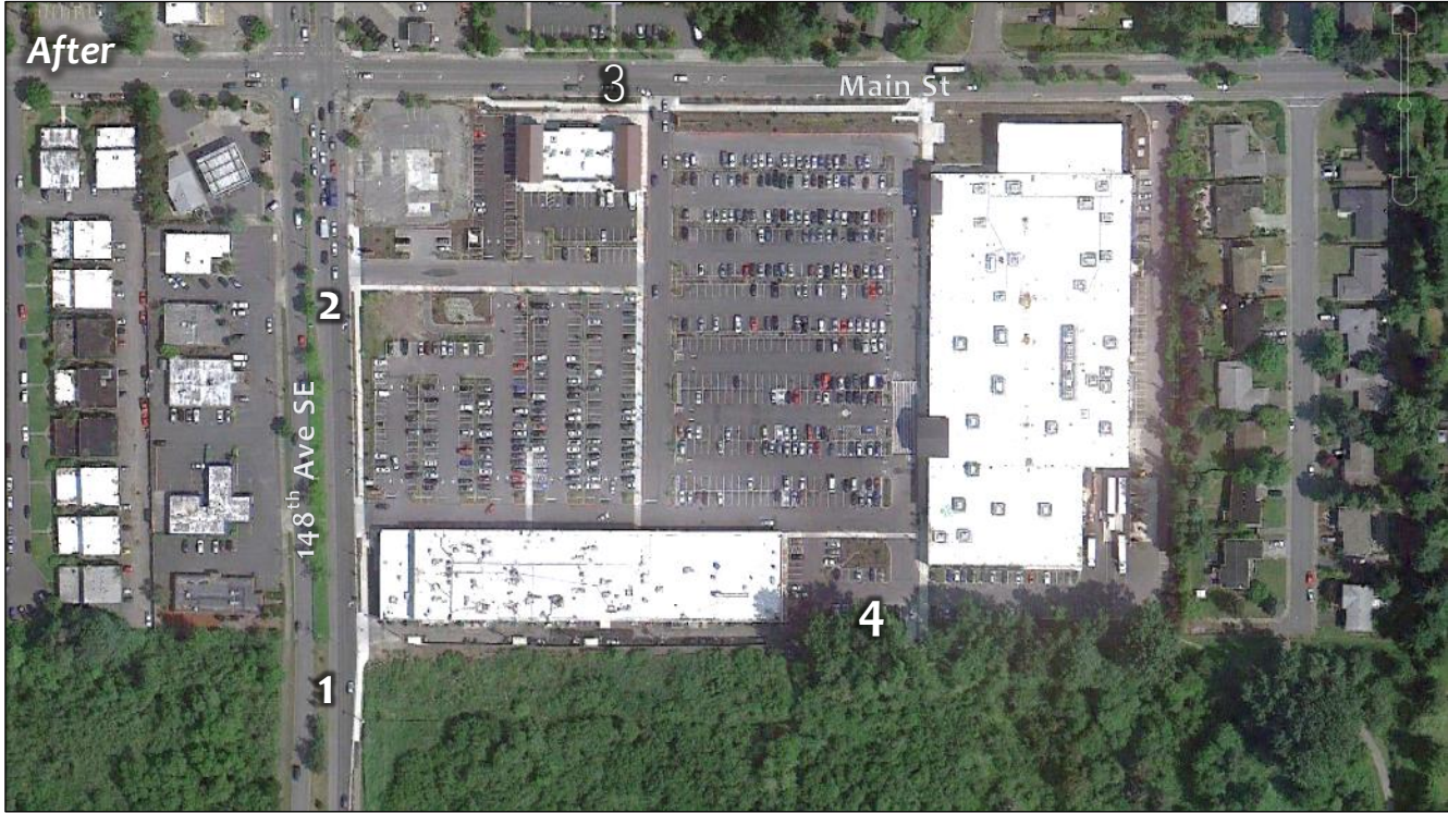
Kelsey Creek Center Aerial Photo
