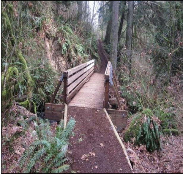
45ft Santa Rosa Glulam Bridge
