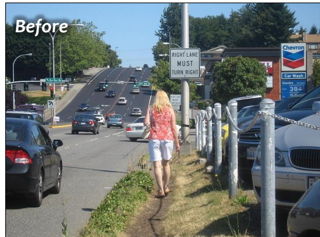
SE 8 th St, just west of Bel-Red Rd, Looking east
