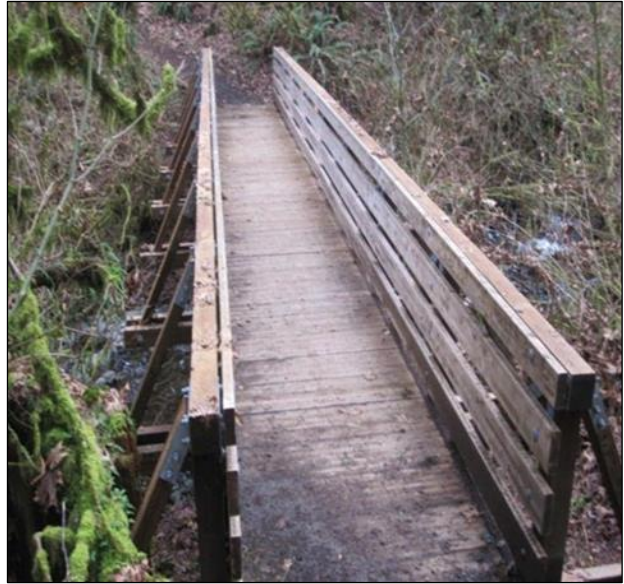
50ft Santa Rosa Glulam Bridge
