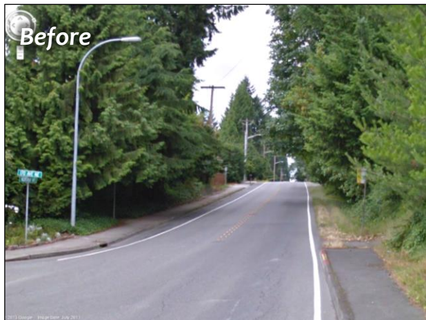
Northrup Way, at 170 th Avenue NE and Northrup Way intersection, looking west
