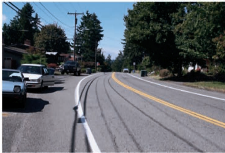
Figure X: Cross Section of Shared Shoulder Facilities Type D: Shared Shoulder with Fog Line (Motor Vehicle Lane + Shoulder \geq 14' )
