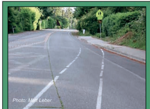
The bicycle lane coming up the hill on 108 th Ave NE stops abruptly, forcing cyclists into the travel lane. This location was identified as an area lacking continuity in the bicycle system.
