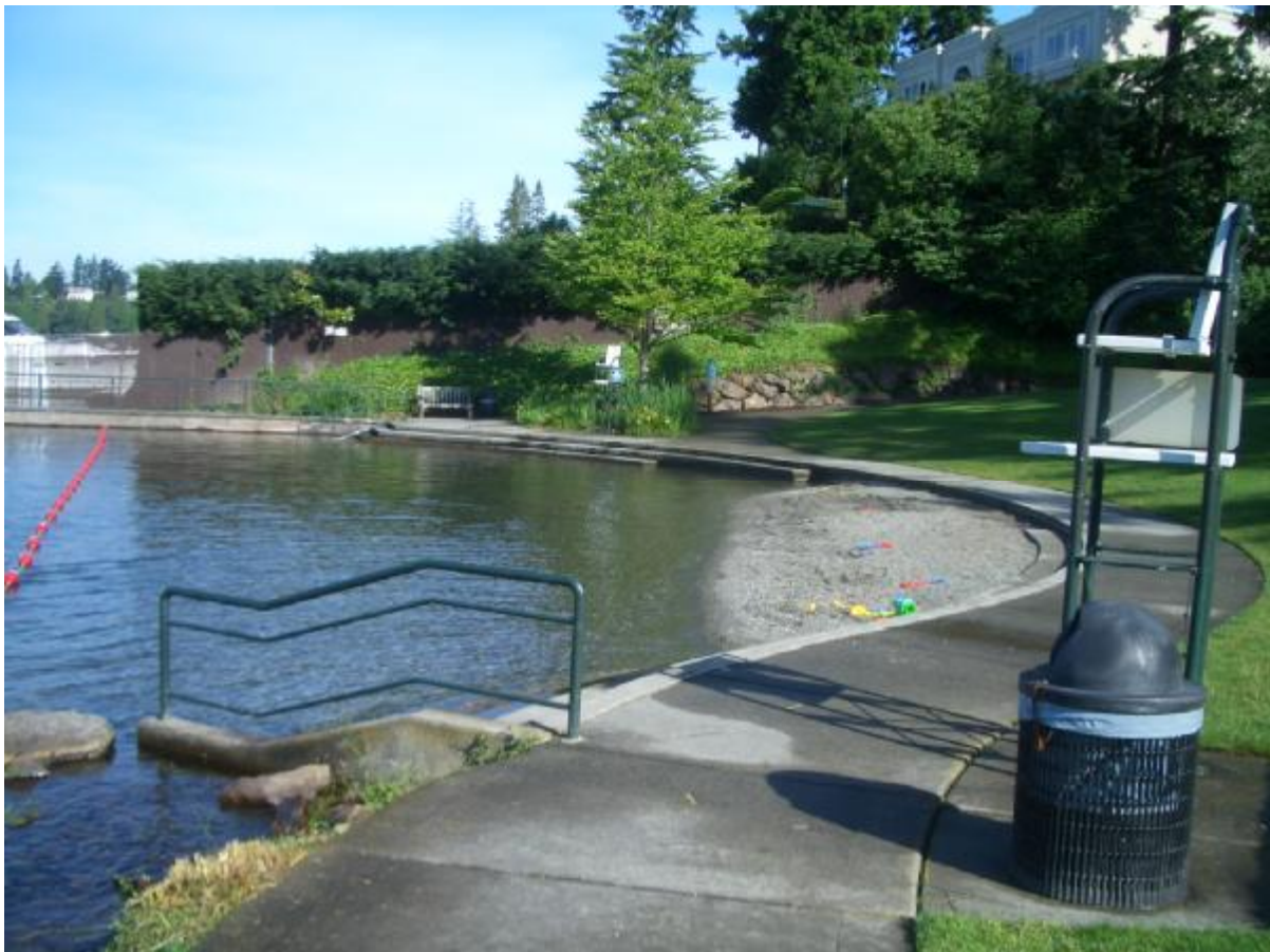
Figure 3. Beach and Concrete Steps at the Swimming Beach (North End)
