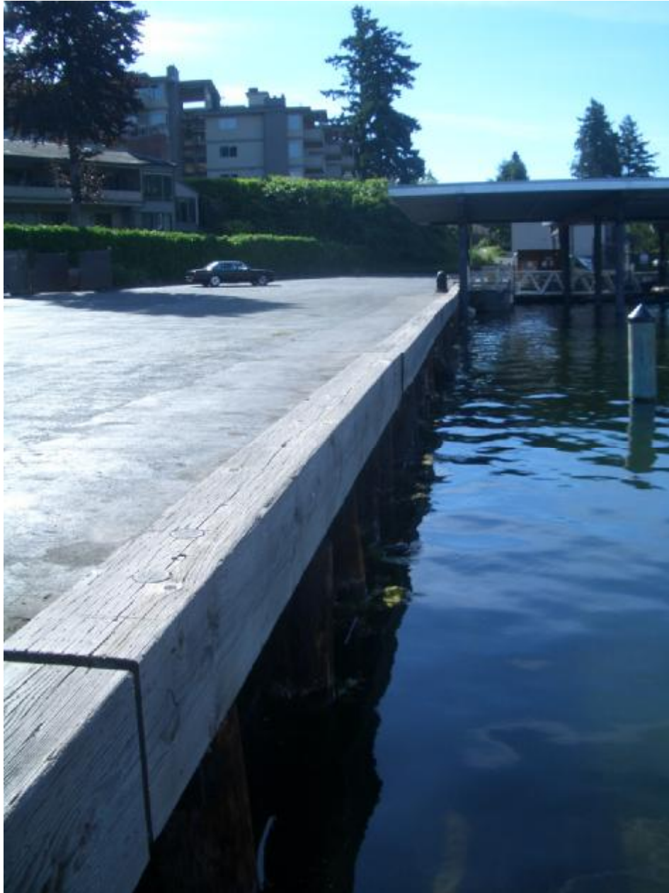
Figure 5: Bulkhead at the Marina
