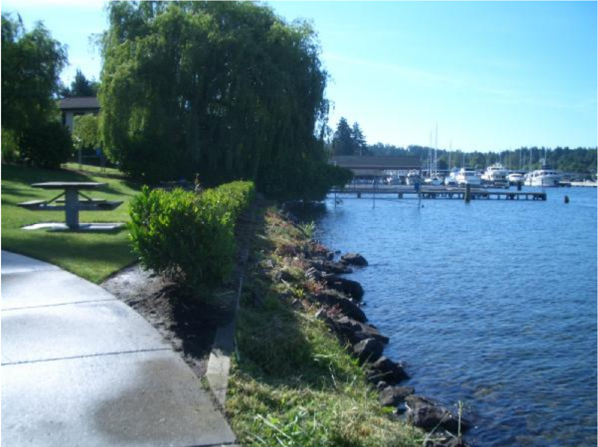
Figure 4. Riprap Slope in the North Central Park Area
