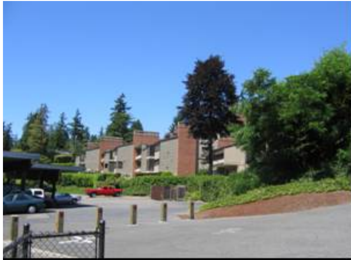
Bellevue Marina Parking Lot and Adjacent Condominiums near 100th Avenue SE
