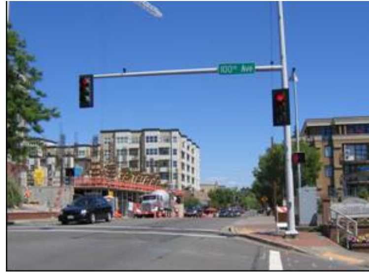
Future Mixed-use Building Under Construction North Side of Main Street
