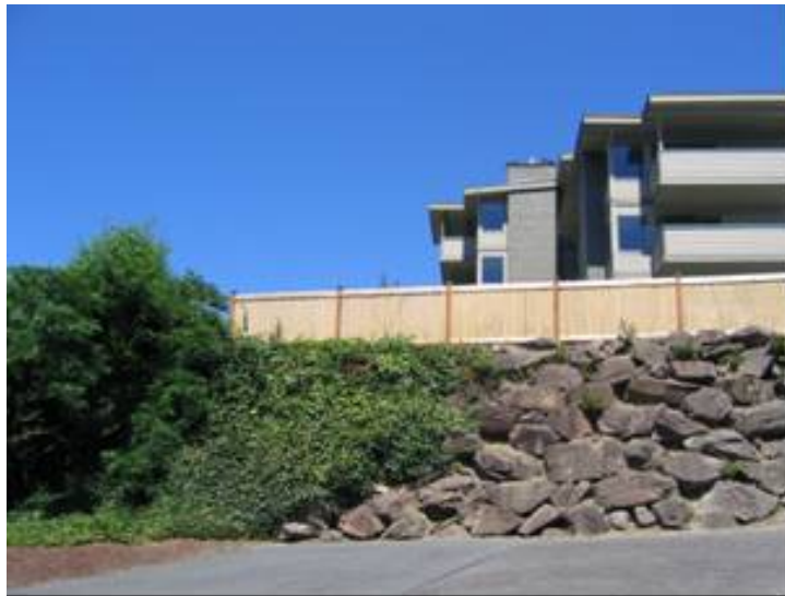
Retaining Wall at Edge of Bellevue Marina Parking Lot
