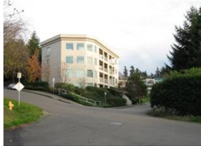
Condominium at Intersection of SE Bellevue Place and Meydenbauer Way SE
