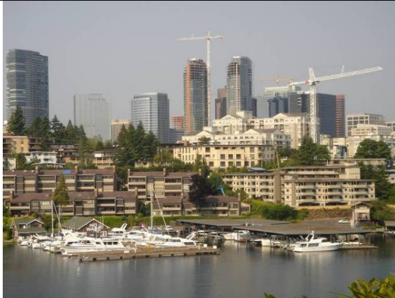
Mix of Residential and Commercial Areas
