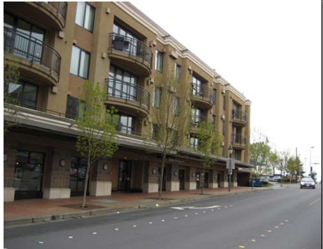
Newer Mixed-Use Structure
