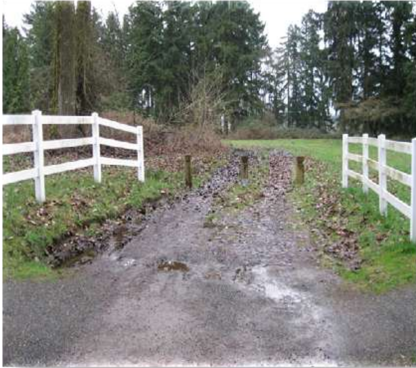
Current 134 th St. Maintenance Access
