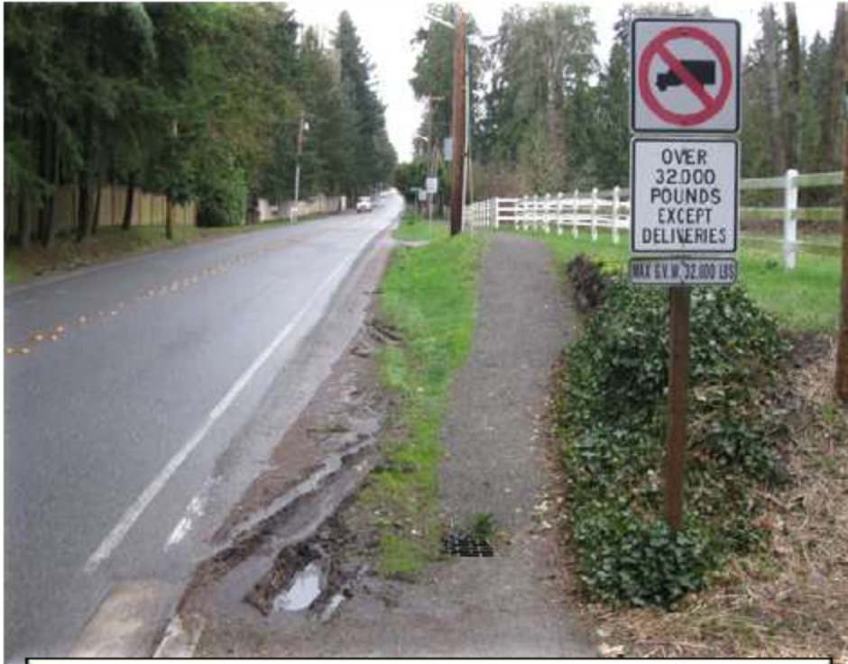
Park Frontage looking North along 134th
