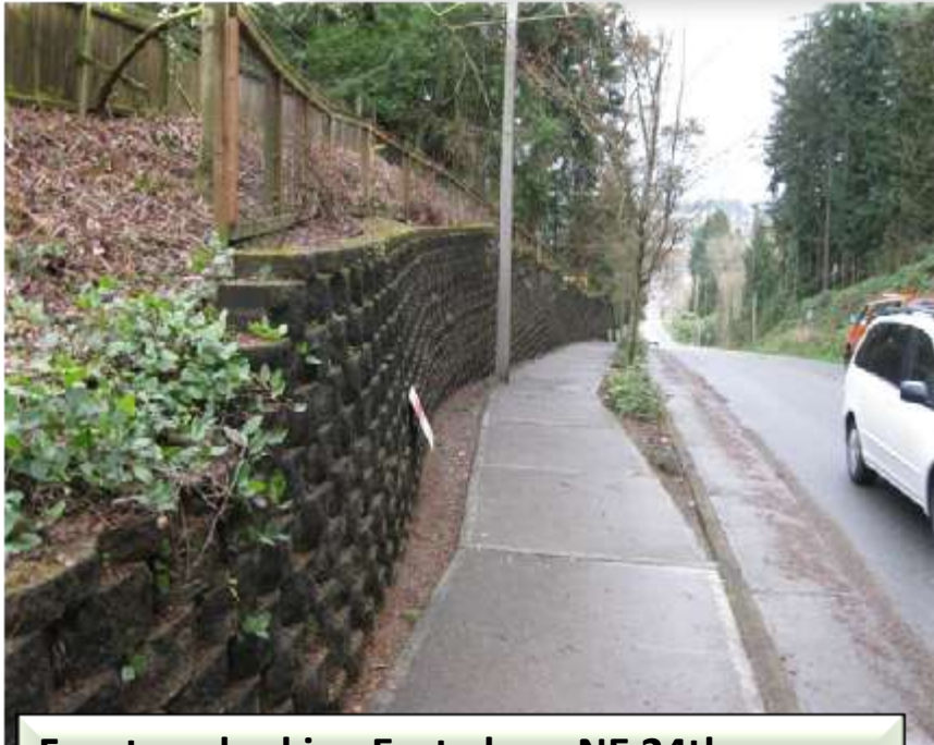
Frontage looking East along NE 24th
