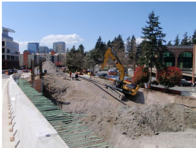
I-405 Utility Relocation at NE 12 th St Overpass
