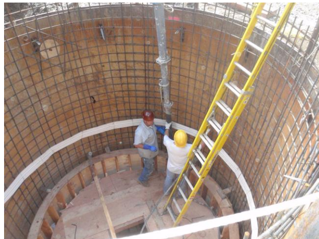
Emerald Ridge Pump Station Construction
