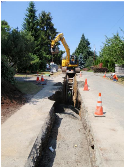
Sewer Service Extension on Cougar Mountain
