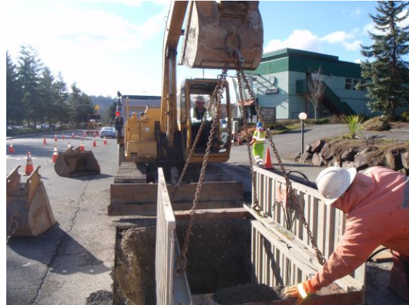
Sewer Repair on 156 th Ave SE
