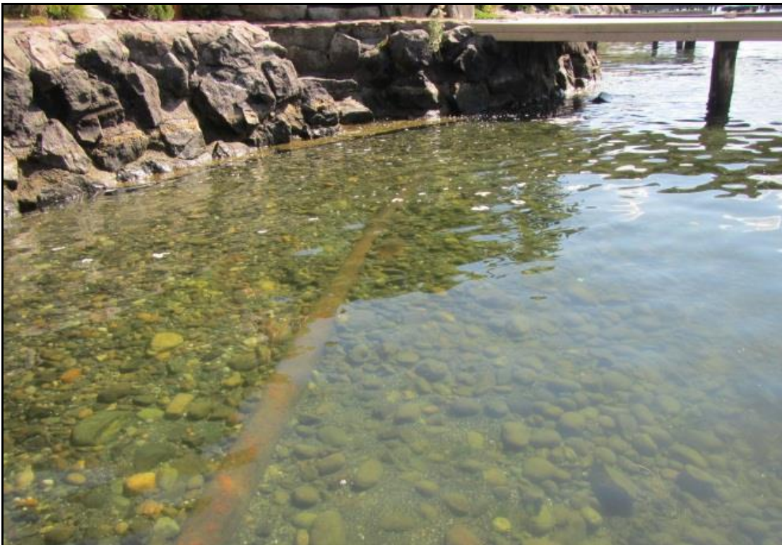
Figure 5-2: Typical View of Exposed Portion of Lake Line Sewer
