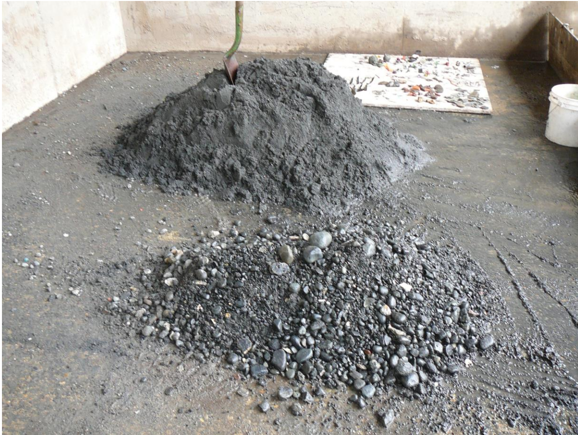
Figure 5-3: Debris Removed from a Portion of Meydenbauer Bay Lake Line Sewer
