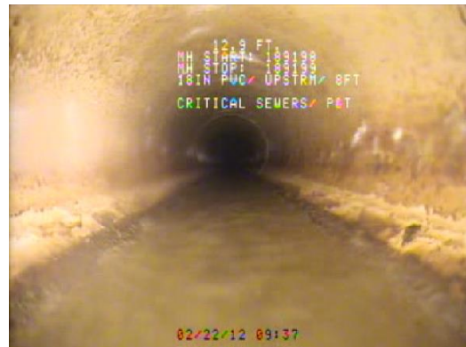
Figure 6-1a: Typical video inspection
