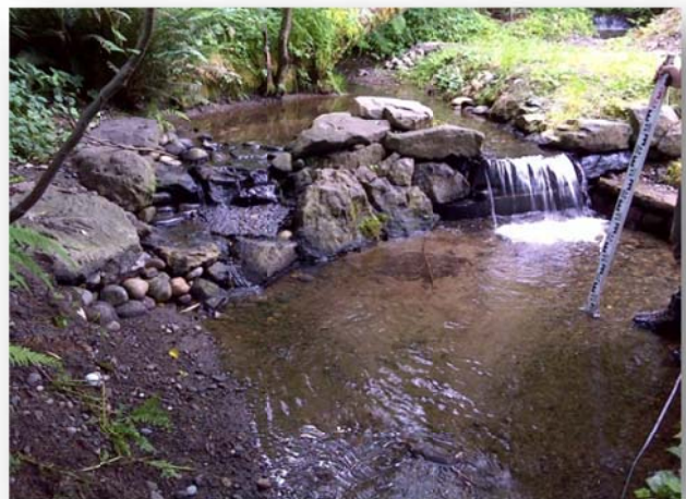
Figure 8. Split Plunge Pool D4 from Constructed Grade Control
