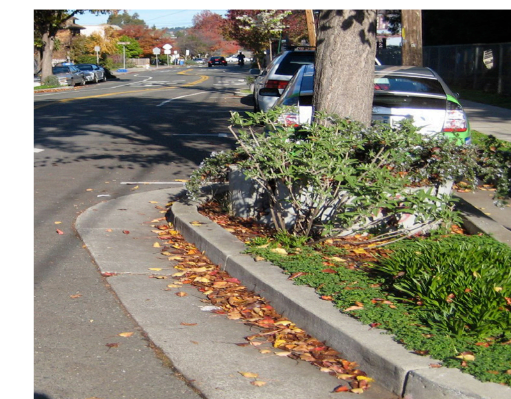
Pinch Point (permanent installation)
