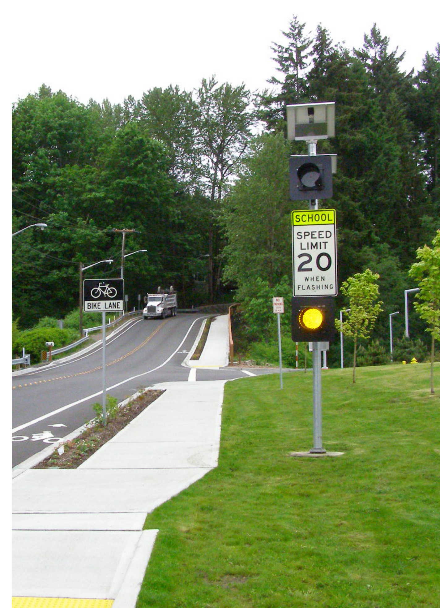
School Zone Sign with Flashing Beacon
