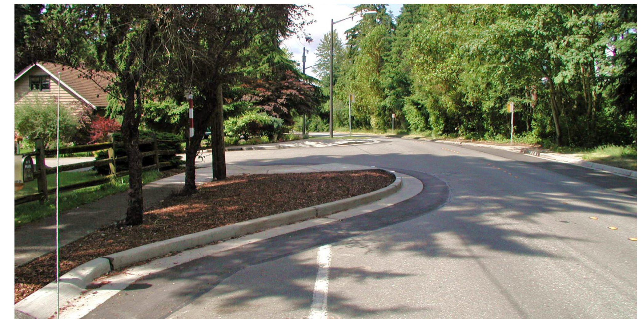
Curb extension at 161st Ave SE
