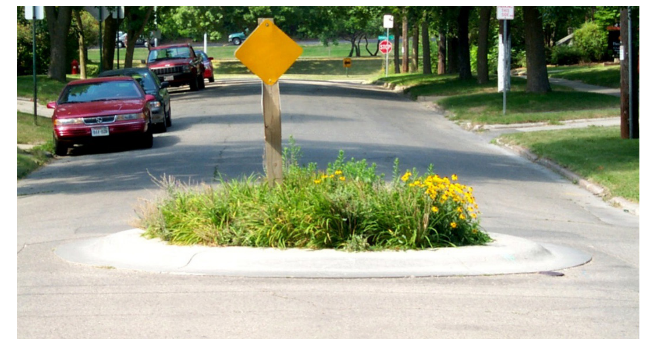
Planted traffic circle
