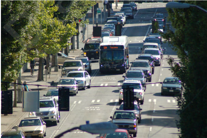
Figure 38 Transit-only lane provides non-curb lane for buses.
