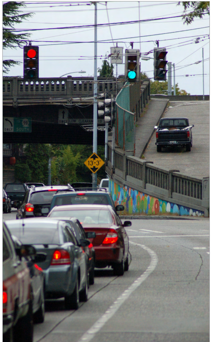
Figure 25 The bus-only queue jump lane (right signal) receives a green signal before general purpose traffic (left signal).
