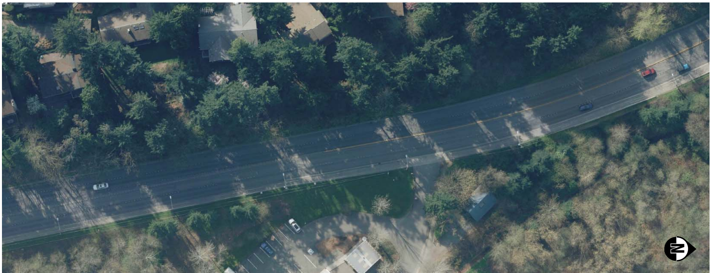
Figure 135 Running Way Improvement Projects L2: A southbound median HOV lane on Bellevue Way SE would improve the speed and reliability of transit vehicles between 112th Ave SE to South Bellevue Park-and-Ride. This would be achieved by constructing one lane on Bellevue Way SE, thereby maintaining all existing general purpose travel lanes. Aerial images depict roadway striping before and after construction.
