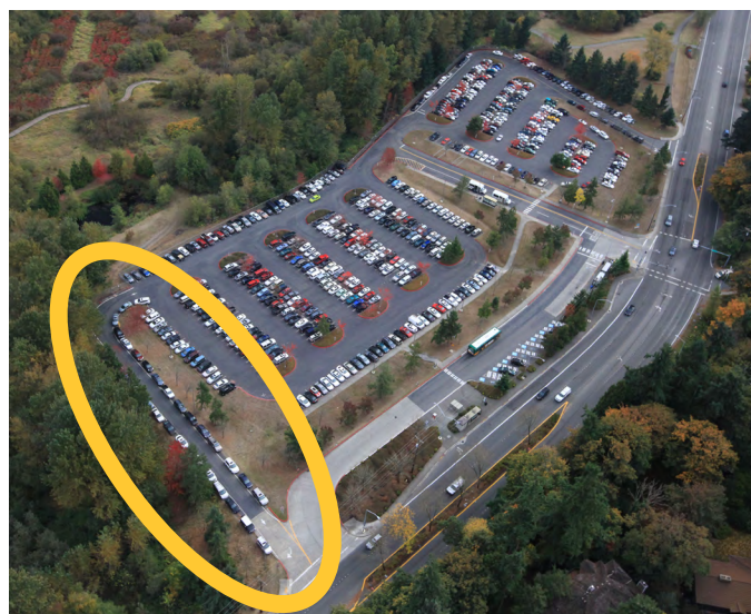
Figure 71 The South Bellevue Park-and-Ride is often over capacity, with vehicles parked along the shoulders of the driveway (circled).
