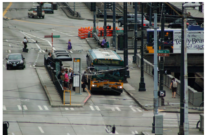
Figure 91 Transit island with bus-only lane.
