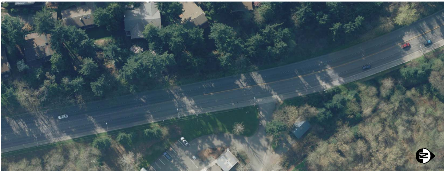
Figure 117 Running Way Improvement Projects L2: A southbound median HOV lane on Bellevue Way SE would improve the speed and reliability of transit vehicles between 112th Ave SE to South Bellevue Park-and-Ride. This would be achieved by constructing one lane on Bellevue Way SE, thereby maintaining all existing general purpose travel lanes. Aerial images depict roadway striping before and after construction.
