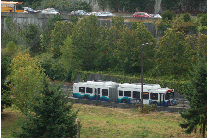
Figure 100 Busways provide dedicated right-of-way for buses.
