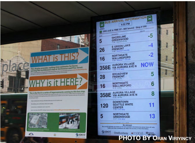
Figure 69 A digital signboard in Downtown Seattle, funded and installed by the Seattle DOT, displaying real-time arrival information from OneBusAway.
