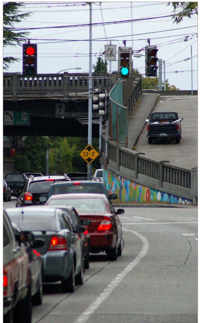
Figure 108 The bus-only queue jump lane (right signal) receives a green signal before general purpose traffic (left signal).
