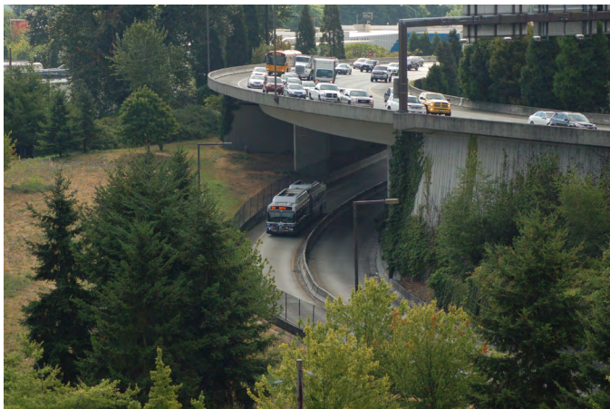
Figure 126 Busways may include grade-separated lanes for buses.
