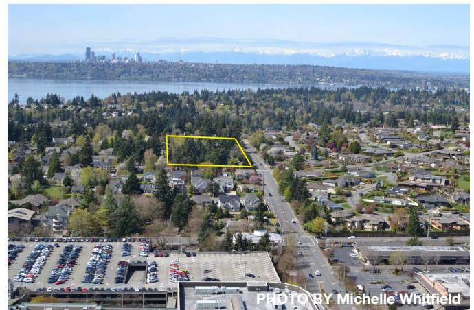
Figure 82 Aerial view of NE 8th St looking west from Downtown, with the Grace Lutheran Church leased park-and-ride lot indicated by the yellow square.
