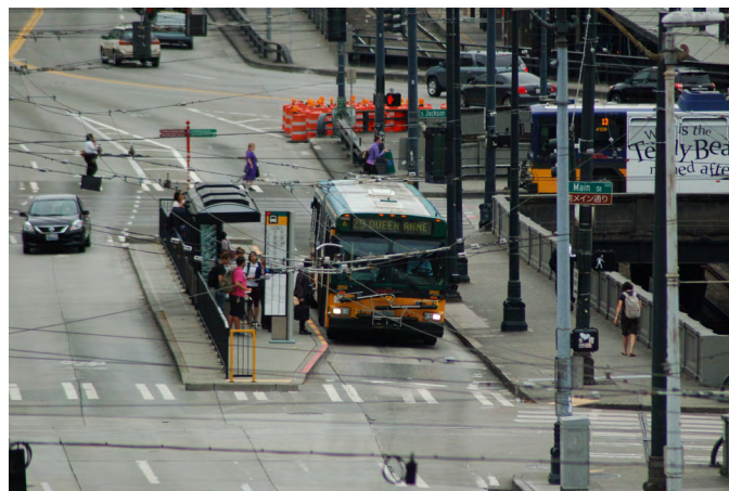
Figure 116 Transit island with bus-only lane.
