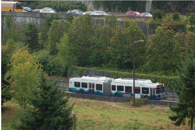
Figure 125 Busways provide dedicated right-of-way for buses.
