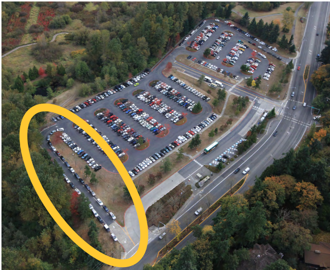
Figure 115 The South Bellevue Park-and-Ride is often over capacity, with many vehicles parked along the shoulders of the driveway (circled).
