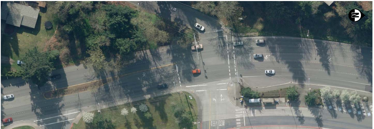
Figure 107 RunningWayImprovementProjectL1: A southbound median HOV lane will be constructed on Bellevue Way SE between the South Bellevue Park-and-Ride and I-90 by Sound Transit as part of the East Link light rail extension project. This will be achieved by constructing a new lane, thereby maintaining all existing general purpose lanes. Aerial images depict roadway striping before and after construction.
