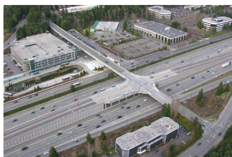
Eastgate Direct Access Ramp (2006) - $19 million
