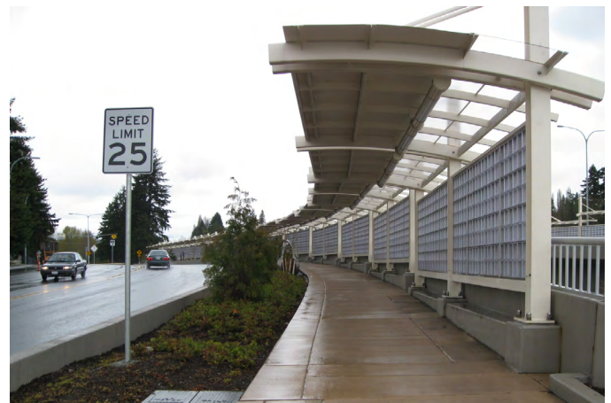
Figure 99 A covered pedestrian walkway at the Totem Lake Freeway Station on I-405 in Kirkland. Similar improvements are envisioned for the Eastgate Park-and-Ride and Freeway Station.
