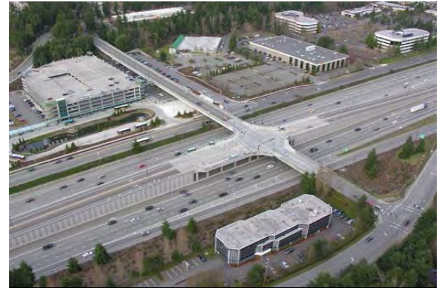
Eastgate Direct Access Ramps
