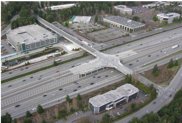
Eastgate Direct Access Ramps
