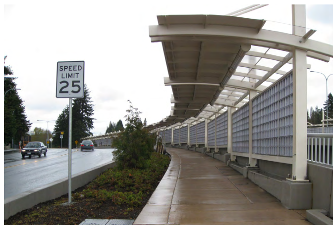
Figure 112 A covered pedestrian walkway at the Totem Lake Freeway Station on I-405 in Kirkland. Similar improvements are envisioned for the Eastgate Park-and-Ride and Freeway Station.
