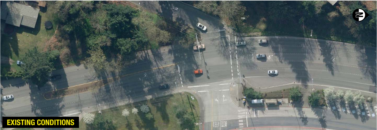
Figure 120 RunningWayImprovementProjectL1: A southbound median HOV lane will be constructed on Bellevue Way SE between the South Bellevue Park-and-Ride and I-90 by Sound Transit as part of the East Link light rail extension project. This will be achieved by constructing a new lane, thereby maintaining all existing general purpose lanes. Aerial images depict roadway striping before and after construction.
