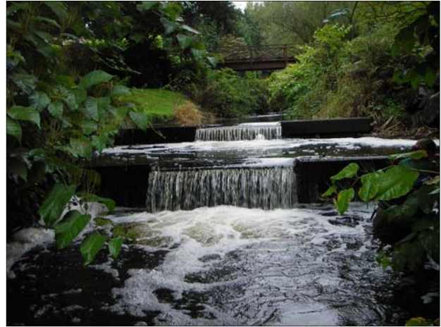
Reach 4: Weirs (September 27, 2010)
