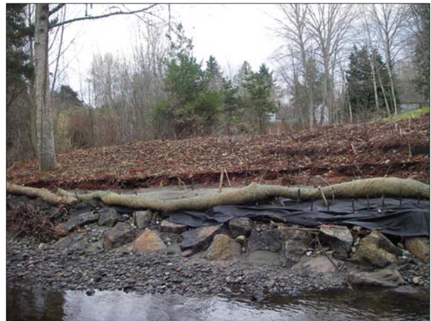
Reach 6: Riparian restoration (September 27, 2010)
