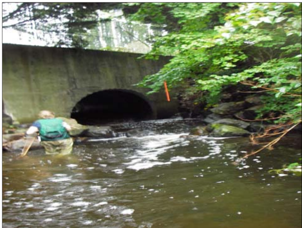
Reach 5: NE 8th culvert (September 27, 2010)
