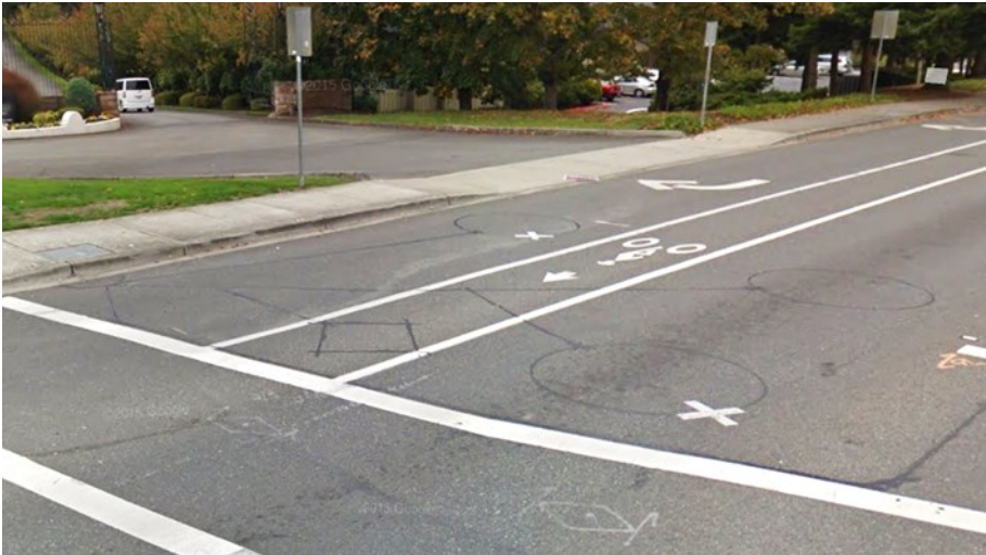
Bike lane inductive loop SE Eastgate Way and 160th Ave SE intersection, westbound
