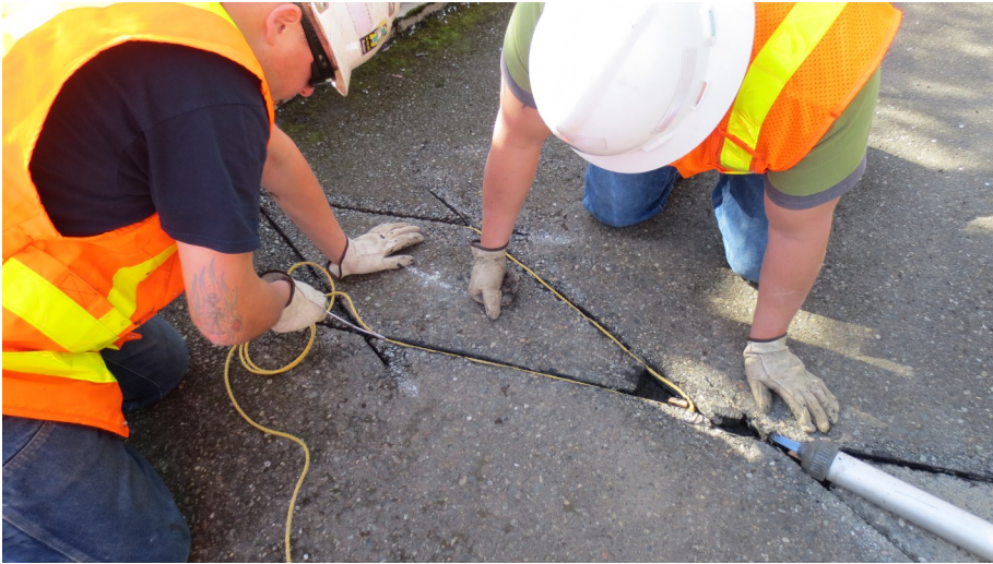
I-90 Trail Counter Installation
