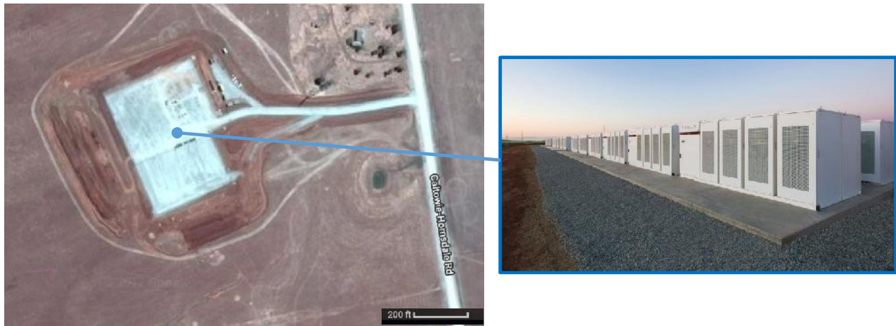
Figure 31: Hornsdale Power Reserve (100MW/129MWh) is approximately 2 hectares in size 83
