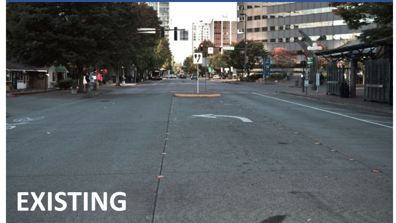
At NE 6th St (Bellevue Transit Center)
