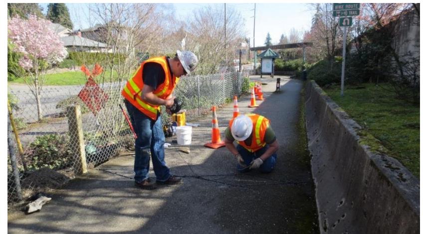
2. I-90 Trail location at SE 34 th St & 109 th Ave SE
