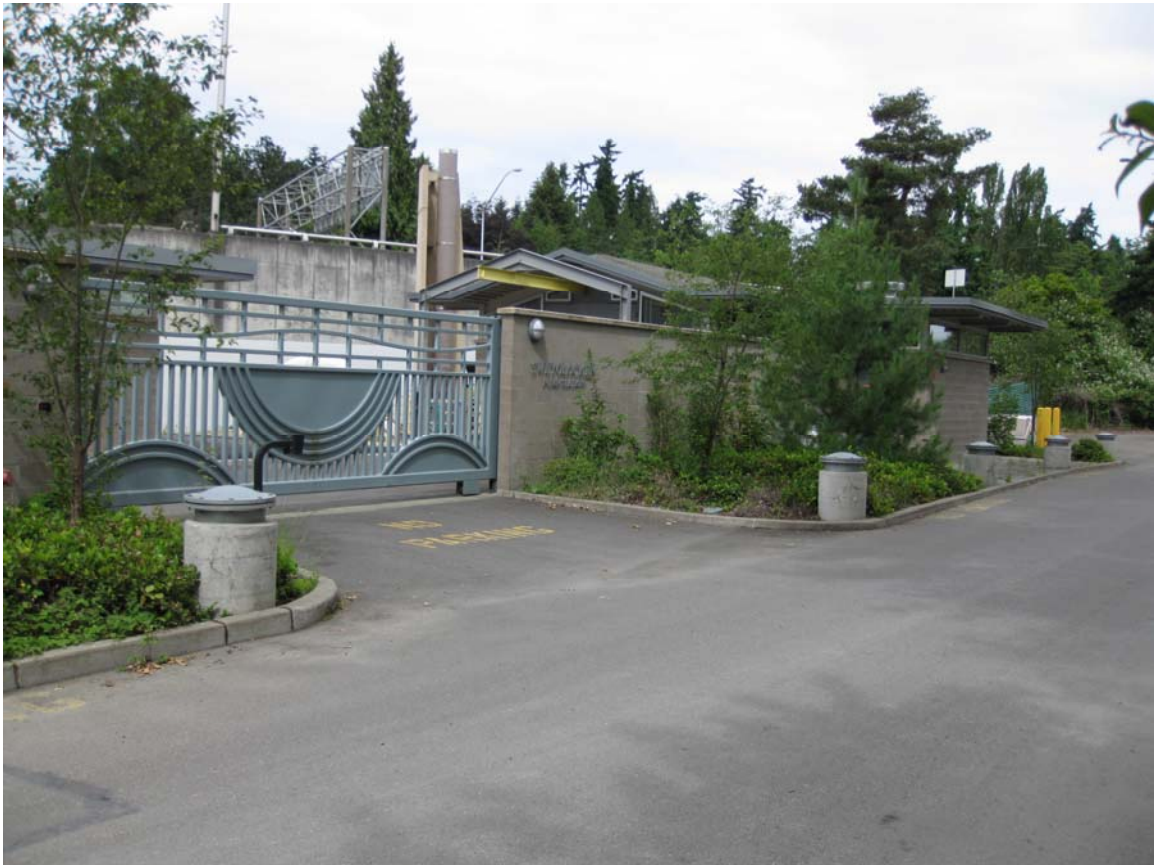
Existing Pump Station
