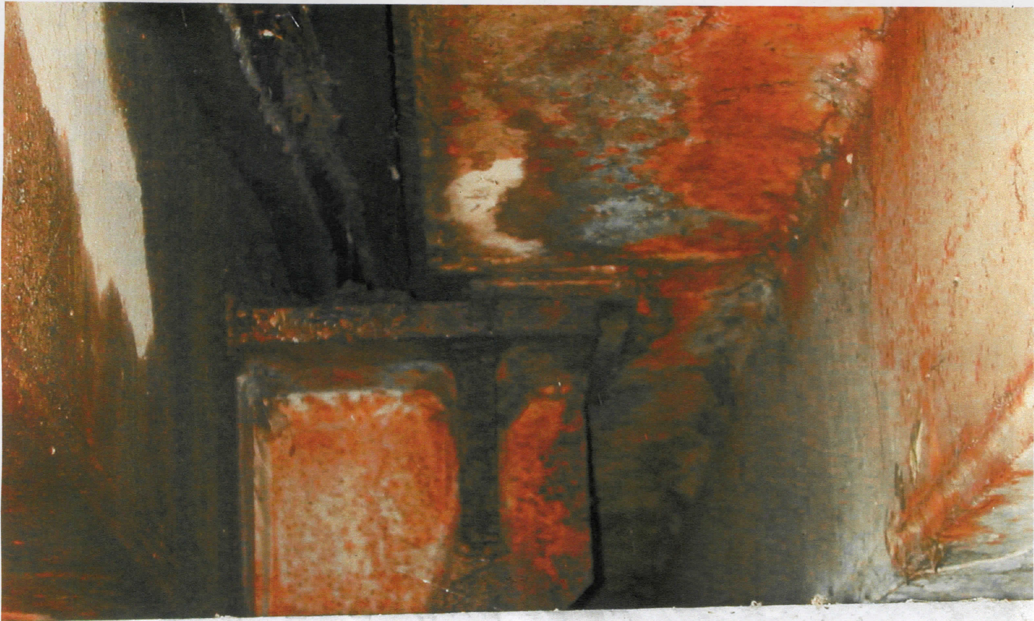
90/43S Bearing F at Joint 2 (near Pier 5) December 2003
