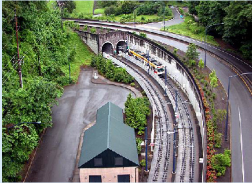
Tunnel portals adjacent to US 26 west of Portland, Oregon
