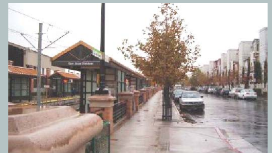
The design and colors of this at-grade station in San Jose integrate the station with the neighborhood.
