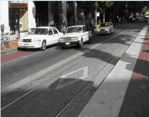
Belgium block trackway on original MAX line in downtown Portland
