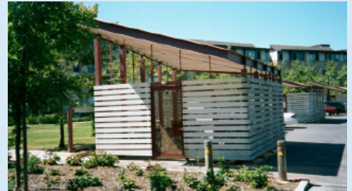
The style of the bike parking structure can be tailored to the neighborhood character.
