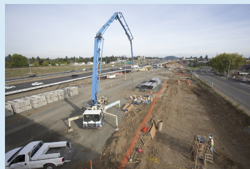
Staging Area, Interstate 205 MAX Extension, Portland. (Damian Conrad Photography)
