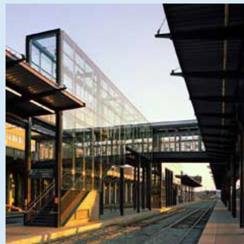
AIA Award winning transit station at King Street Station in Seattle.
