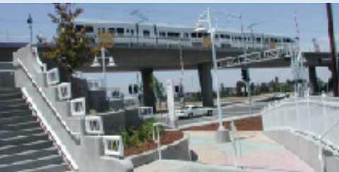
Elevated VTA track - The open design of this VTA track maximizes visibility while employing urban design elements such as pedestrian-scale infrastructure. Transit users are more likely to feel safe in this environment.
