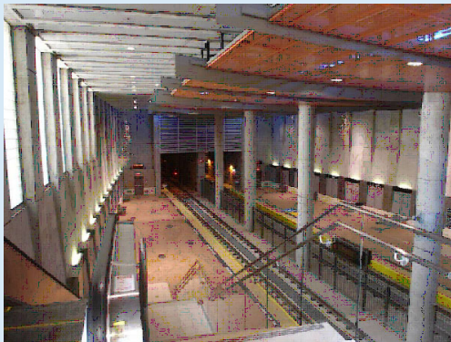
The safety of this underground station in San Diego is enhanced by natural light, high quality stonework, transparent materials, pedestrian scale architecture and exquisite maintenance. The transparent upper level of this structure is at the street level – so pedestrians on the street can observe activities in the underground station. This offers additional security for those inside.
