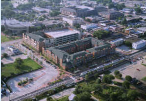
DART station and TOD in downtown Plano - TOD in Addison, Texas near the Addison DART Station
