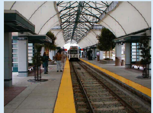
This suburban San Jose station is integrated into the surrounding neighborhood through the use of colored paving, plantings, and benches. The structure offers protection from weather, while capturing natural light and using open architecture with clear sight lines.
