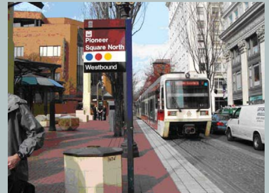
At-grade light rail system through downtown at Pioneer Square Station. TriMet uses Belgium block in downtown rail application because it is durable and easy to replace.
