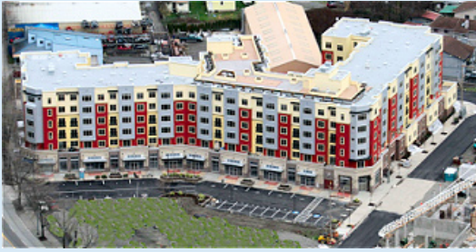
Courtland Place Rainier Court in Seattle - Development like the Courtland Place has sprung up along a light rail line in Seattle that won't operate until 2009.
