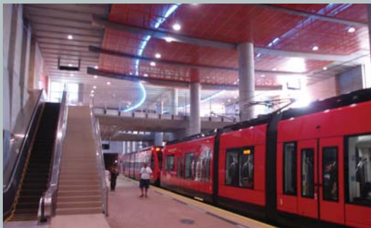
The San Diego State University tunnel employs design features including natural light and air, high quality finishes, and art to create a comfortable waiting environment.
