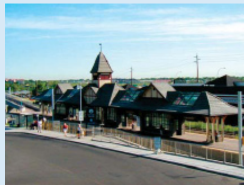
Fish Creek/Lacombe Station in Calgary - The City of Calgary has encouraged TOD in part through an effort to minimize roadblocks to good developers.
