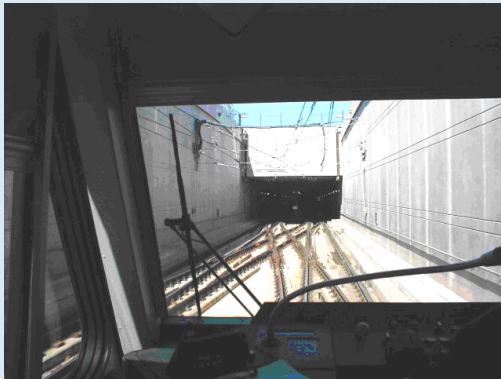
Cut and cover tunnel portal in Dallas, Texas
