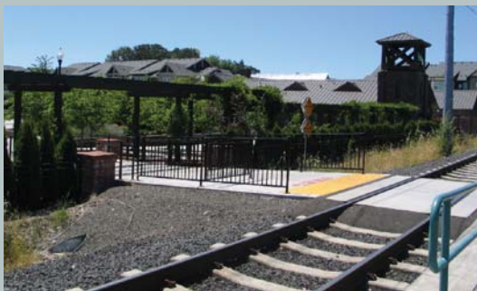
Pathway connects Orenco Gardens, a multi- and single-family development with Orenco Station.
