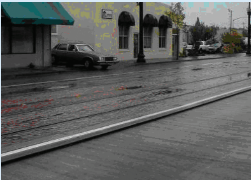
Mountable trackway of colored and stamped concrete, Hillsboro, Oregon
