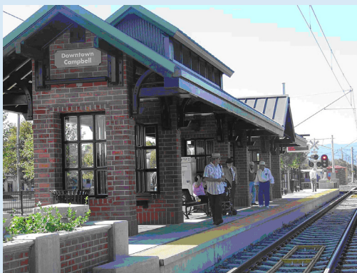
Raised platforms at light rail transit stations provide an easier and safer entry onto the light rail line (VTA, Campbell, CA).
