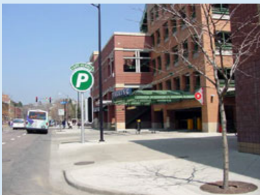
Public parking wrapped in commercial uses in Boulder, Colorado - Parking structures in the City of Boulder are often wrapped in commercial uses, as shown here. Efforts in Boulder are also made to ensure that parking structures materials and design fit with the general architectural style of the area.
