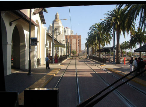
San Diego Trolley Station - This station uses architectural detailing that is consistent with the surrounding community, which enhances a sense of area identity.
