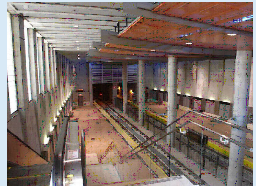
Underground station at San Diego State University
