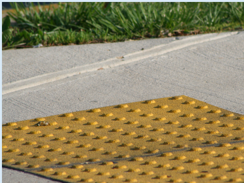
Two examples of tactile warning strips for visually impaired people (Flickr sources: Darrin Frazer above and Clearly Ambiguous below).
