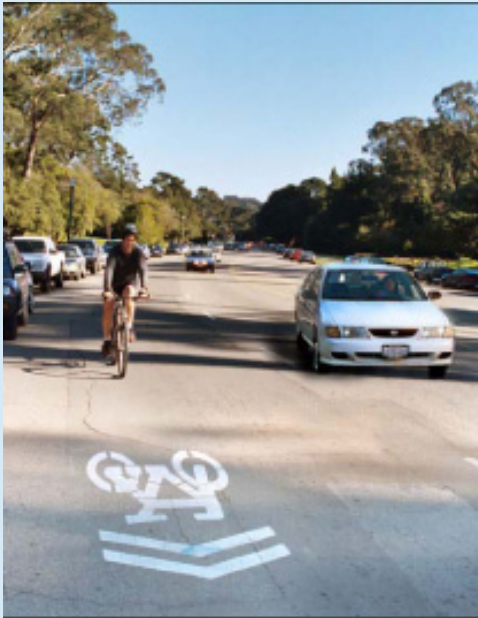
Sharrows painted in lieu of a bicycle lane along JFK Boulevard through San Francisco's Golden Gate Park (Source: San Francisco Department of Parking and Traffic report entitled, "San Francisco's Shared Lane Pavement Markings").
