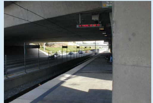
Underpass stations that are dark or have hidden areas are more likely to have higher crime rates.
