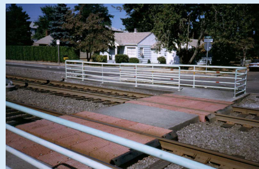
Z-crossing in Portland, Oregon - The Z-crossing is one method of creating safe pedestrian and bicycle crossings.
