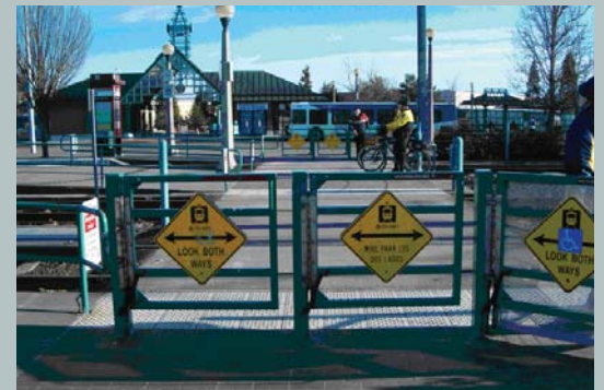
Pedestrian signage at track crossing and security presence at Beaverton Transit Center.
