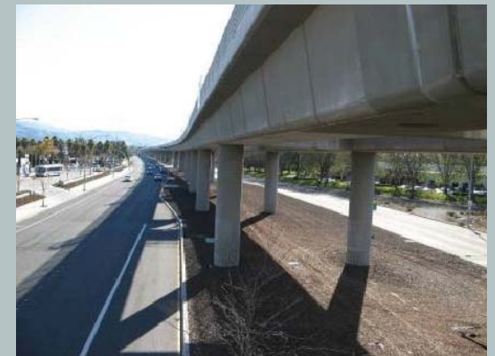
Elevated trackway in San Jose.
