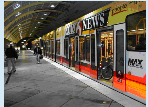
Underground station serving two-car light rail trains in Portland, Oregon
