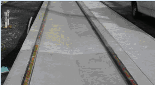
Paved concrete track installation on Portland Interstate MAX.
