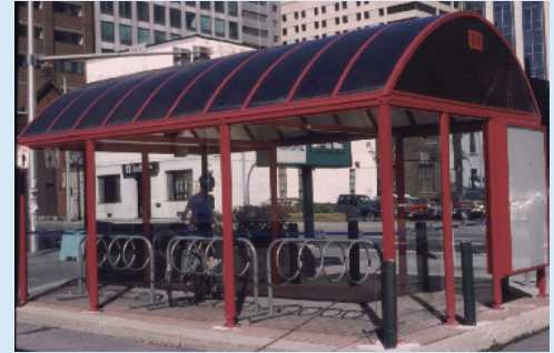
Bike parking at stations should be protected from poor weather and in plain view to prevent theft (note glass enclosure above).
