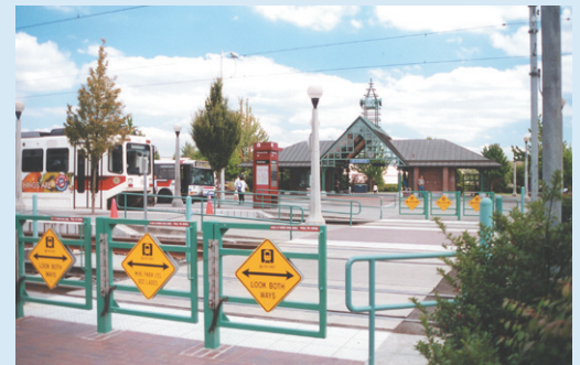
Pedestrian safety gates installed after a fatality at Beaverton Transit Center, a busy transit center serving buses and Portland MAX. These gates provide access for autos and pedestrians to the adjacent commercial and residential communities.
