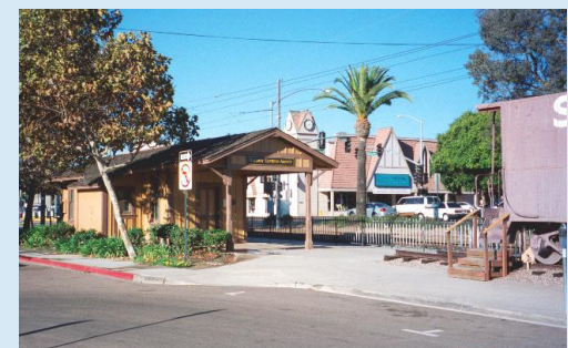
Small community station adjacent to single family neighborhood in San Diego.
