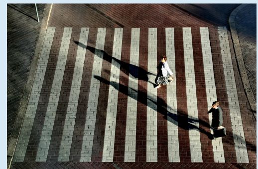
A zebra crossing in Helsinki, Finland (Flickr source: La Febbra).
