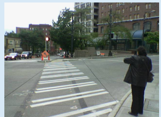
This zebra crossing at 3rd Street and Yesler in Seattle has a wide turning radius that permits vehicles to turn the corner at unsafe speeds, endangering pedestrians (Flickr source: Joe Goldberg).
