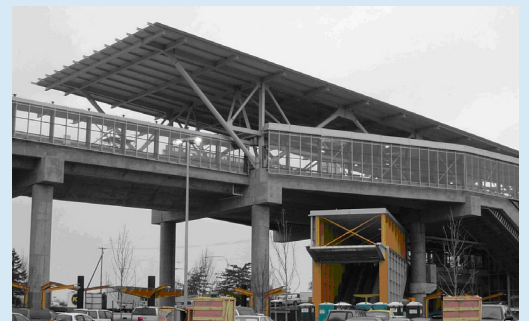
Elevated station construction Seattle (Tukwila)
