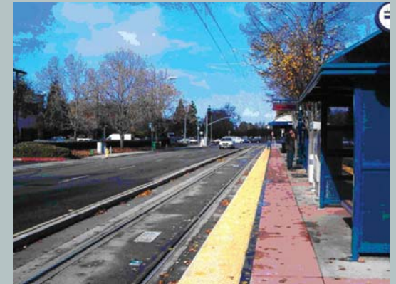
Street configuration and tactile curbs in San Jose.
