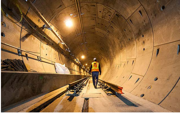
Tunnel for One Light Rail Track
