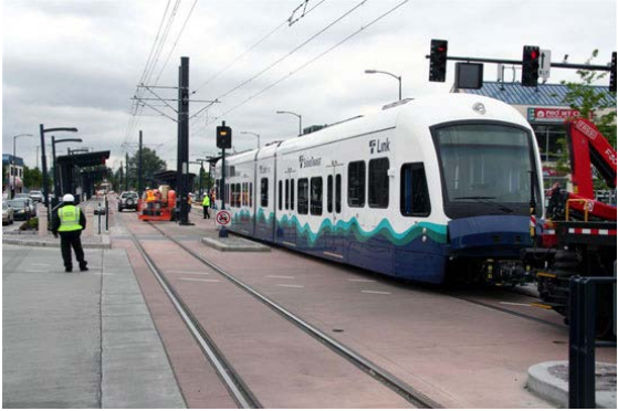
Light Rail Catenary System
