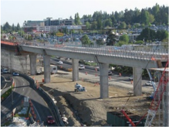
Elevated Light Rail Guideway
