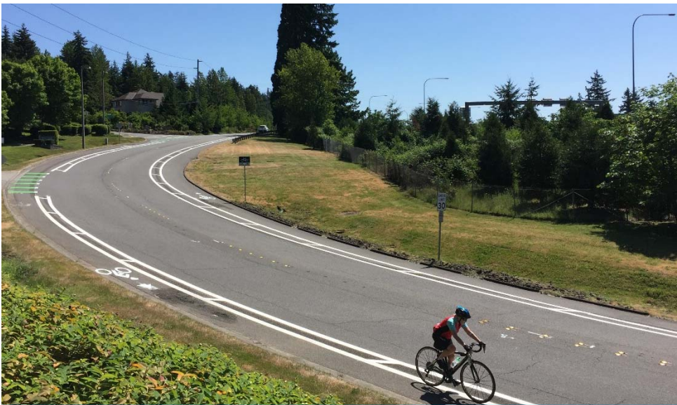
NE 24 th Bike Lane Project-after
