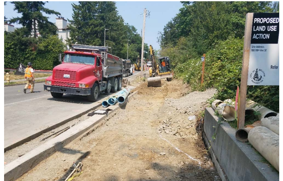
118 th Ave SE Sidewalk-during
