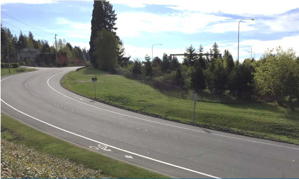
NE 24 th Bike Lane Project-before
