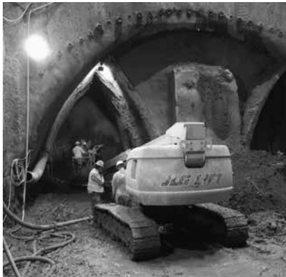
East Link trenching Page 3
