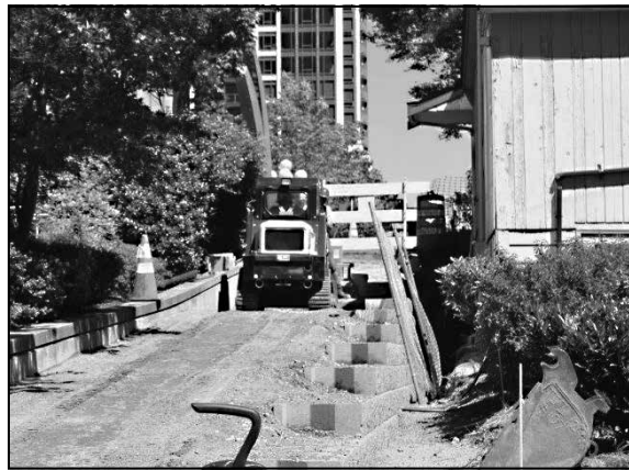
The Northeast Sixth Street pedestrian corridor, sometimes called the “cattle chute,” is being widened and given a more gradual incline.
