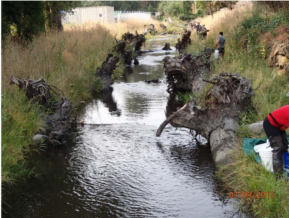
Photo 9. Richards Creek, RM 0.15 and grade/erosion control structures composed of large woody debris
