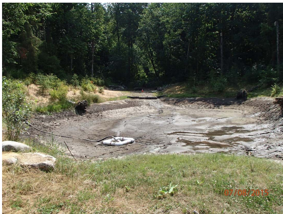
Photo 7 Anna's Pond, engineered for high flow bypass and sedimentation adjacent to Coal Creek survey reach, RM 1.3
