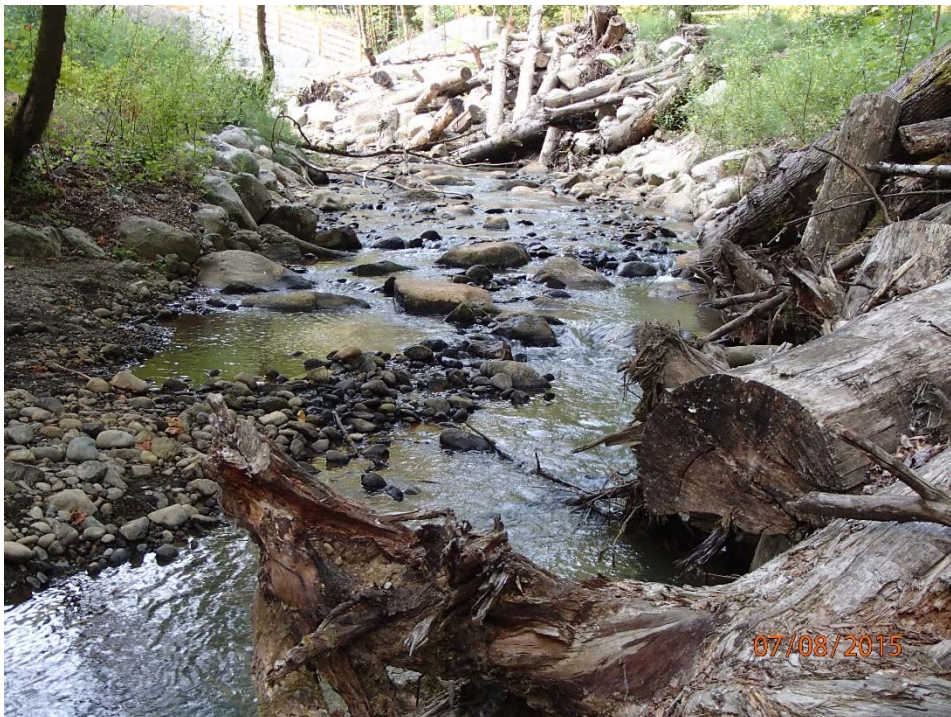
Photo 2. Engineered log jams for habitat and bank stability at Coal Creek, RM 1.8 below Coal Creek Parkway
