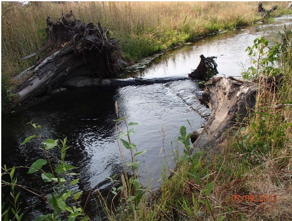
Photo 10. Individual grade/erosion control structure on Richards Creek, RM 0.15
