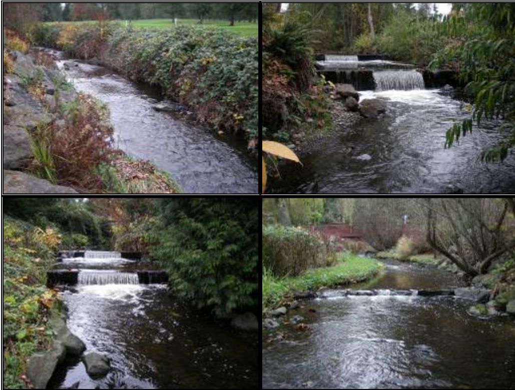
Figure 26. Typical habitat in Reach 5.
