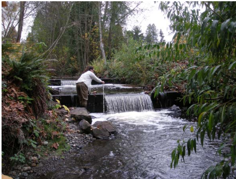
Figure 20. A photo of the concrete grade-control weir in Reach 5 that may have been a partial migration barrier in 2007.
