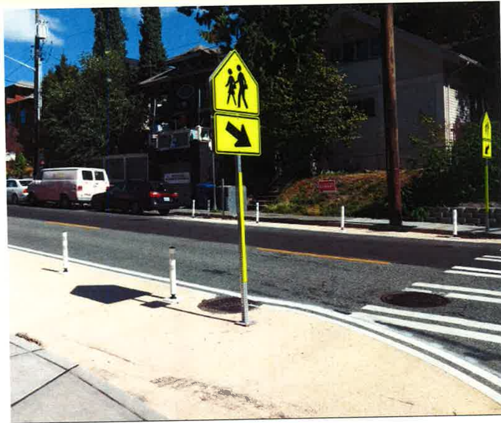
Painted shoulder Separated from Travel Lane by Painted Stripe and Posts
