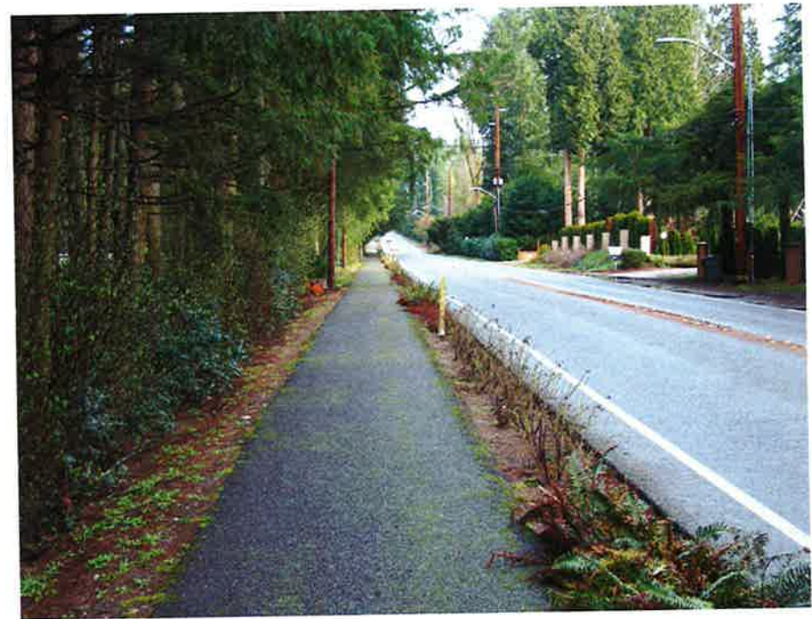
Asphalt Path Separated from Travel Lane by Planter Strip
