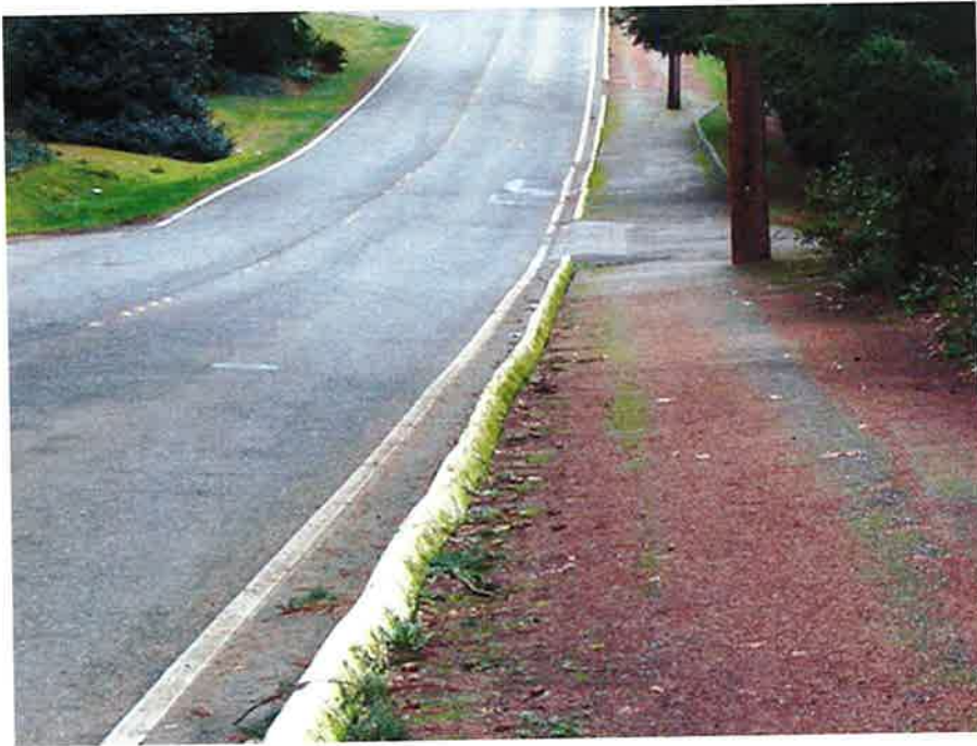
Asphalt Path Separated from Travel Lane by Curb
