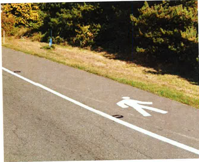
Shoulder Separated from Travel Lane by Painted Stripe
