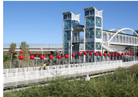
The 142nd street bridge is improved with sculptural wayfinding elements and marks entry to Eastgate
