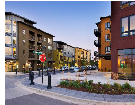
An improved east-west "main street" ties BC, P&R, residences, and offices together with activity hub
