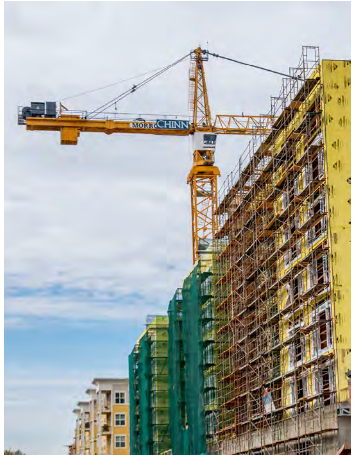
Construction in Redmond
