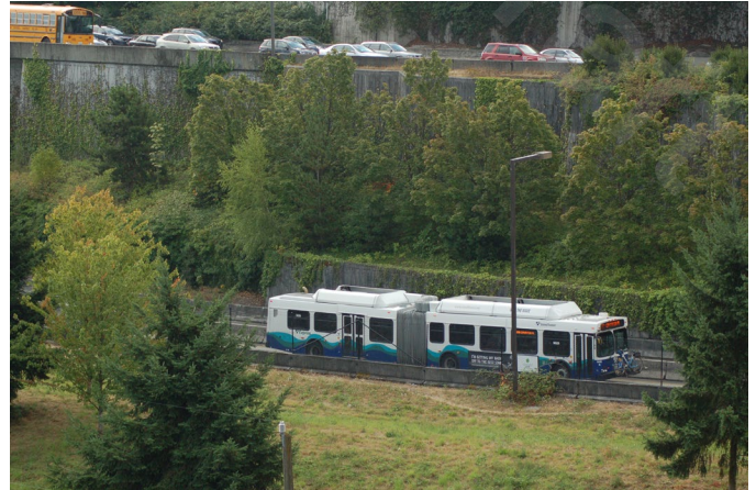
Figure 41 Busways provide dedicated right-of-way for buses.
