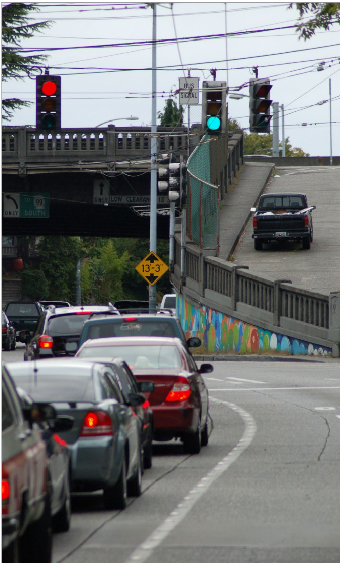
Figure 24 The bus-only queue jump lane (right signal) receives a green signal before general purpose traffic (left signal).
