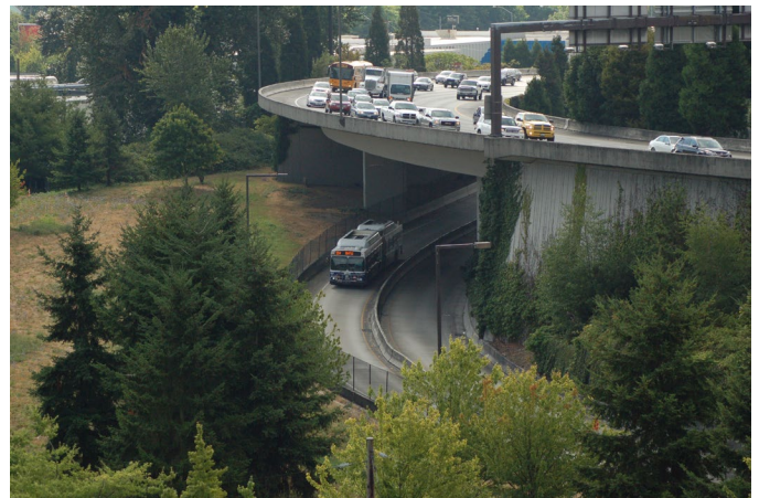
Figure 42 Busways may include grade-separated lanes for buses.
