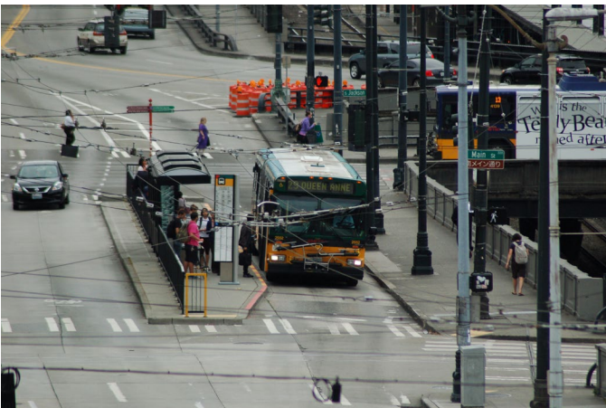
Figure 32 Transit island with bus-only lane.
