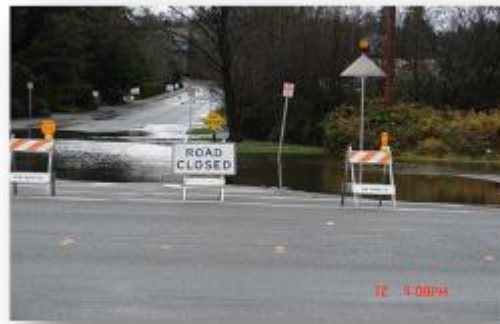
Figure 6-9. NE 21st Street floods on December 12, 2010.
