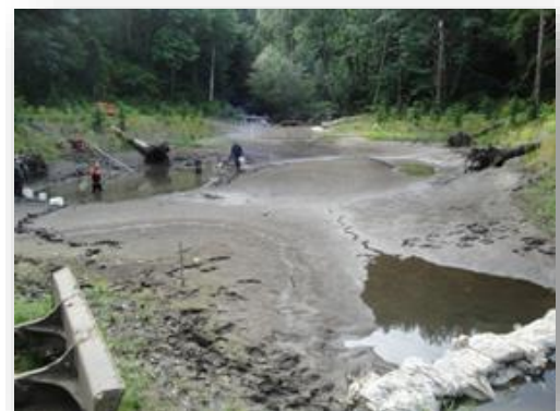
This photo shows the Coal Creek off-channel sediment pond, ready for sediment removal.
