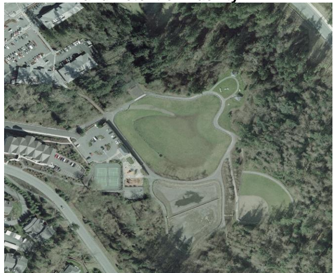
Lakemont Stormwater Filtration and Detention Facility
