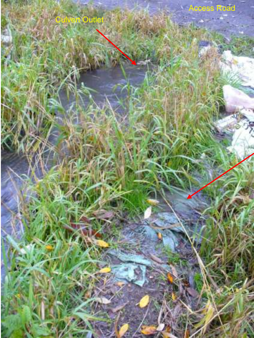
Photo 13 – Following moderately rainy weather, water is spilling out of the channel just downstream of the culvert crossing. 11/26/18
