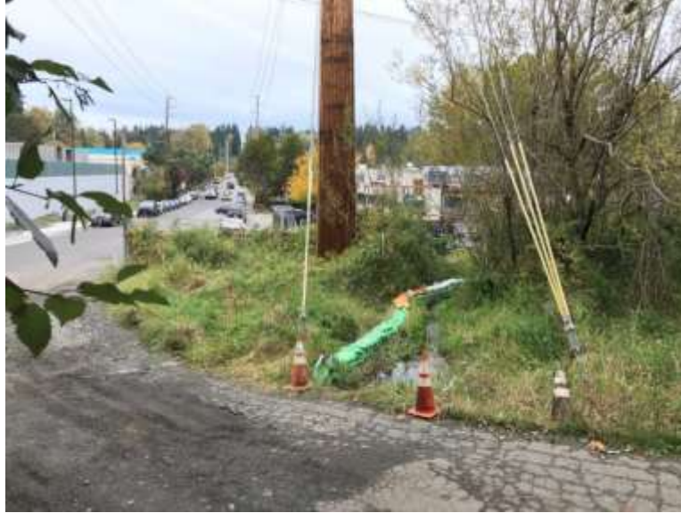
Photo 8 – Downstream from the access road showing the proximity to SE 30th Street on the left side of the photo. Flows which jump the ill-defined channel upstream (behind the photographer) do not re-enter the stream but rather end up in the SE 30th storm drainage system, or on the street surface if the drains are overwhelmed. 10/19/16
