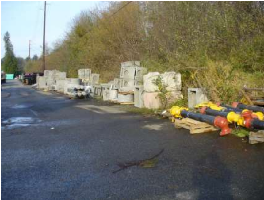
Photo 11 – Western project area boundary along the Fowler storage yard. Note the perpetually wet pavement due to seepage from the stream, which is perched higher than the yard along this section. 11/20/18
