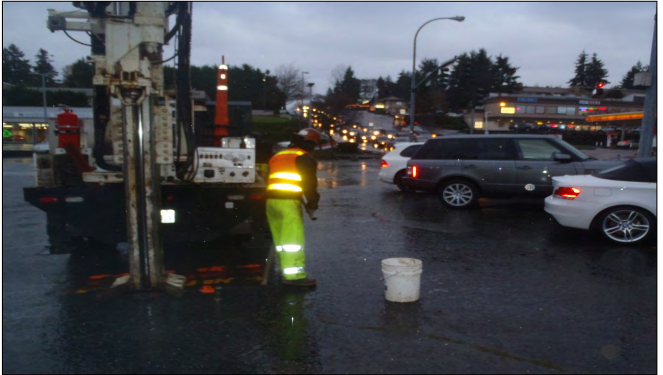
Drilling at Triangle Lot Property for B-116E boring – Looking East
