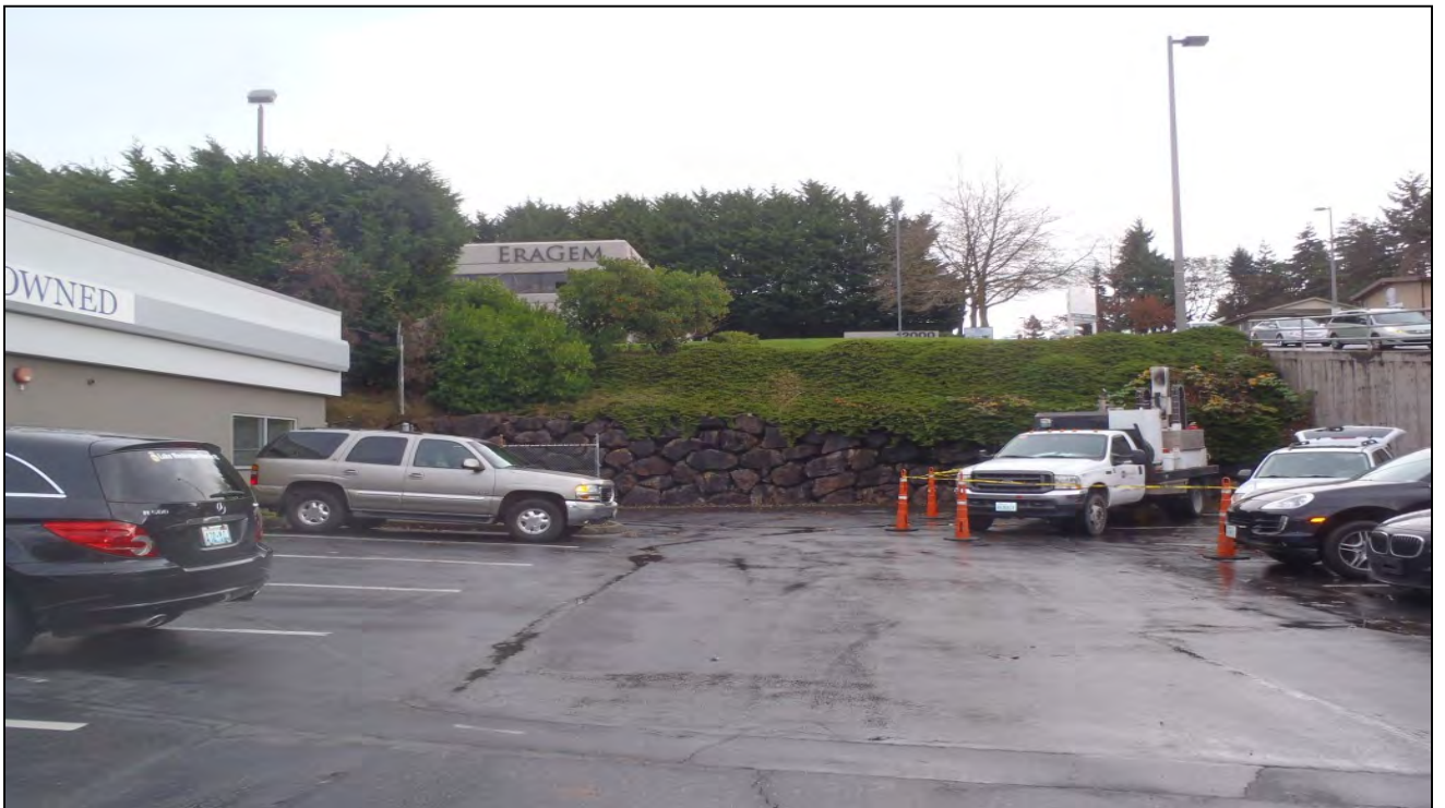
Drilling at the Bakker property to complete B-115E boring – Looking East
