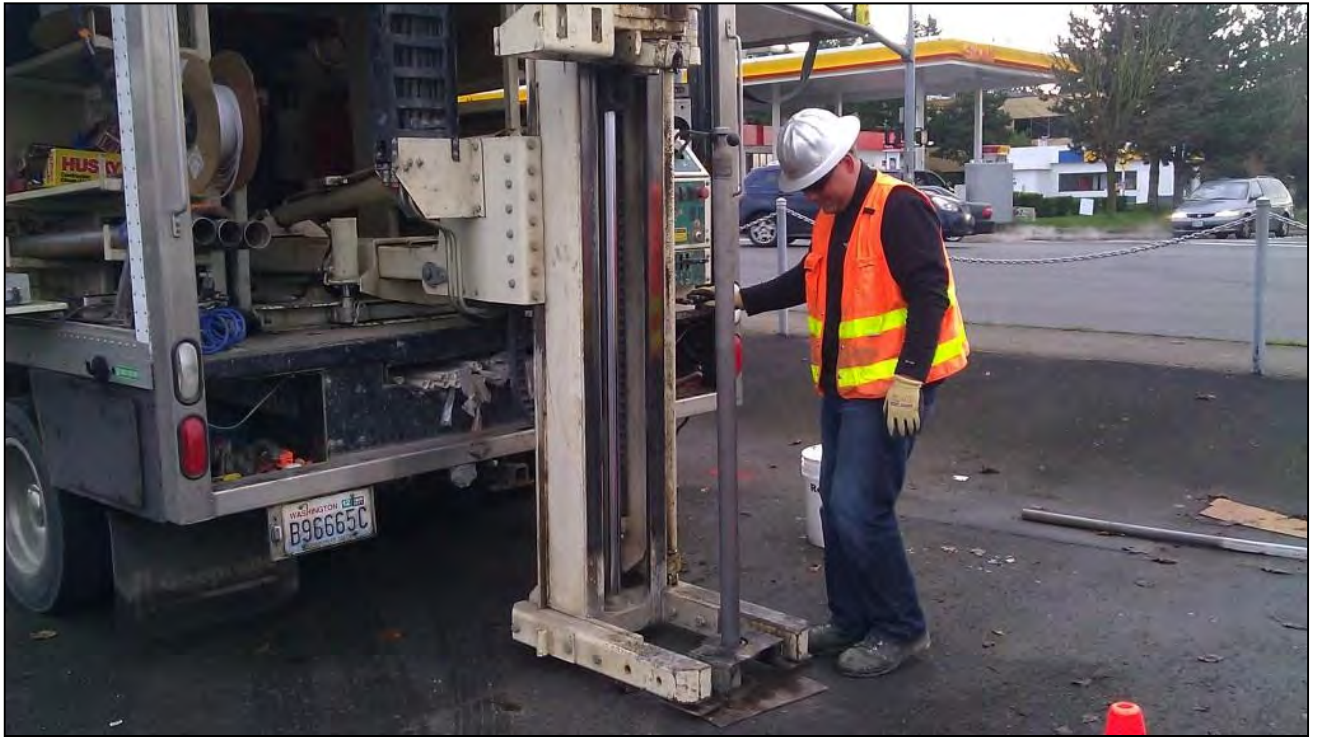
Direct-Push drilling activities to perform boring B-104E – Looking Southeast
