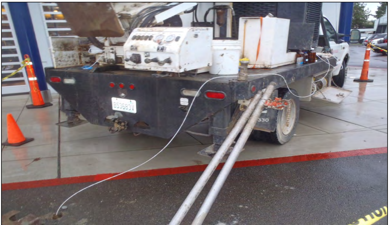
Groundwater sampling from B-119E exploration – Looking East
