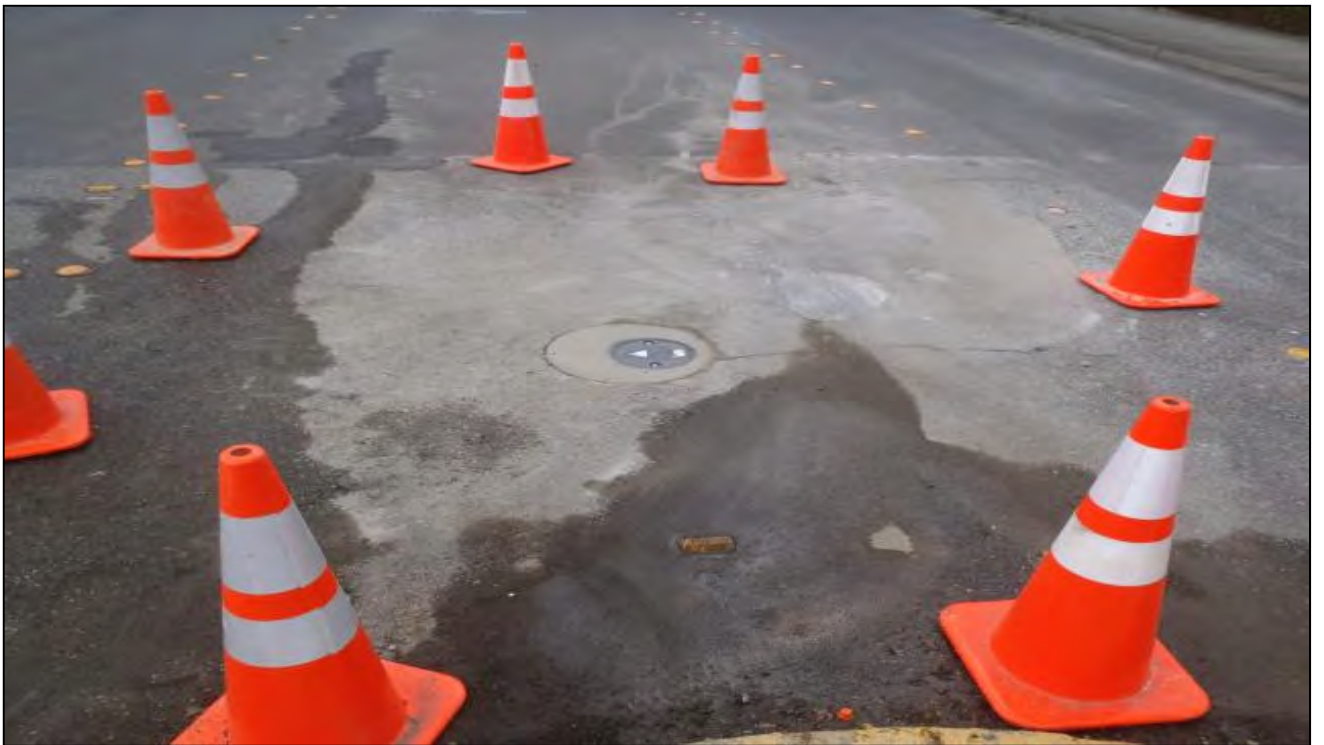
Completed monitoring well with monument installed, typical
