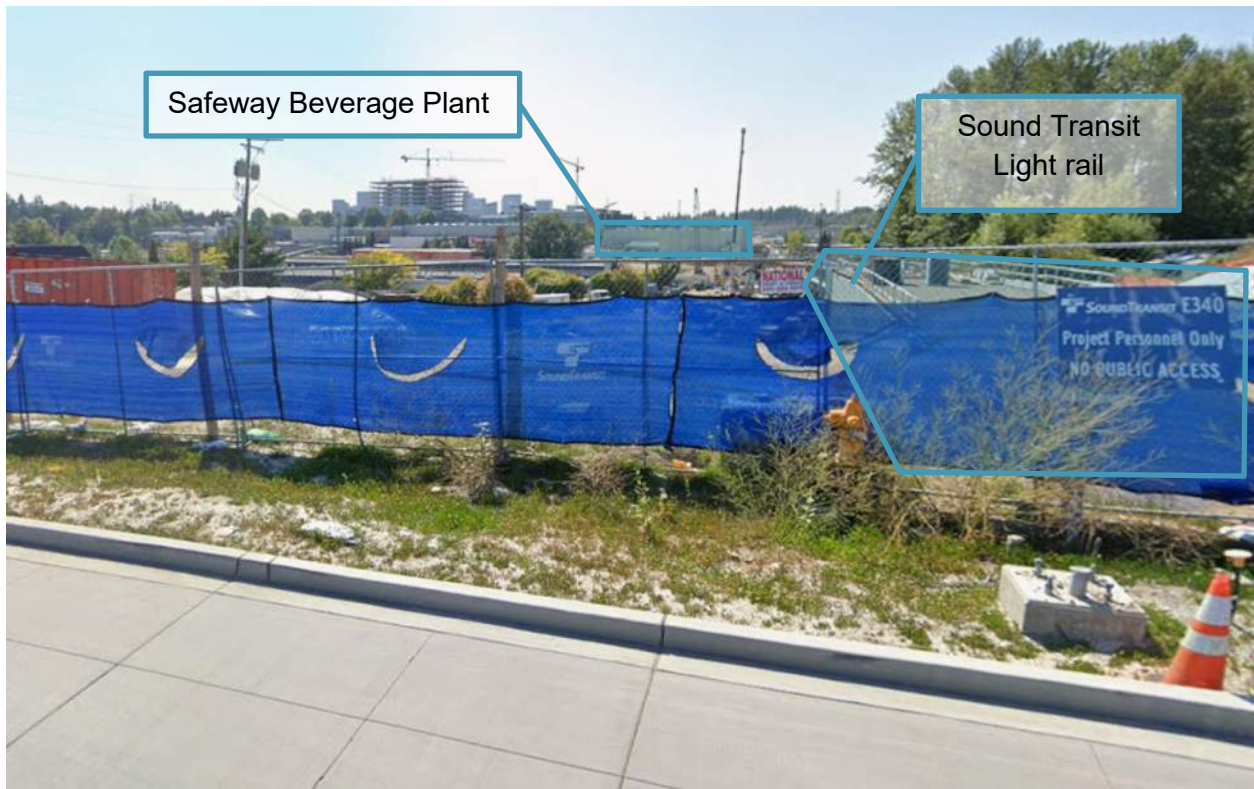
Figure 3 – Existing Condition Street View, 130 th Ave NE Area D, Looking West
