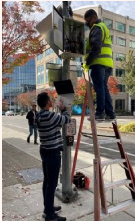
Figure 9: Staff install Cellular Vehicle-to-Everything (C-V2X) equipment in Bellevue
