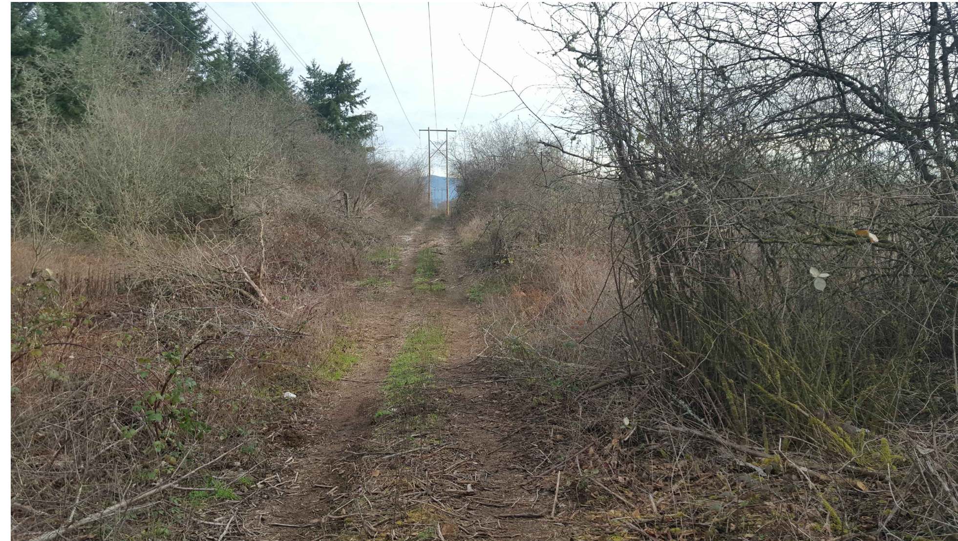
A PUGET SOUND ENERGY RIGHT OF WAY MAINTENANCE PATH THROUGH LOW GROWING SHRUBS AND TREES.
