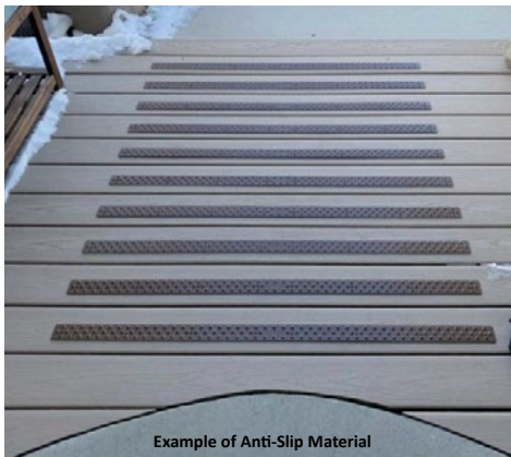
Example of Anti-Slip Material
