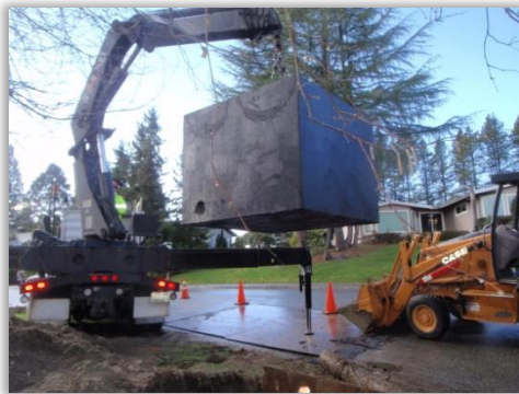
PRV Vault Replacement
