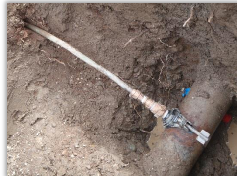
New Service Line and Saddle
