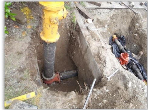
Fire Hydrant Replacement
