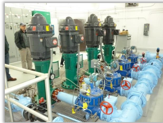
Newport Pump Station Rehabilitation
