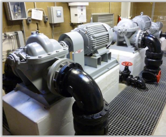
Woodridge Pump Station
