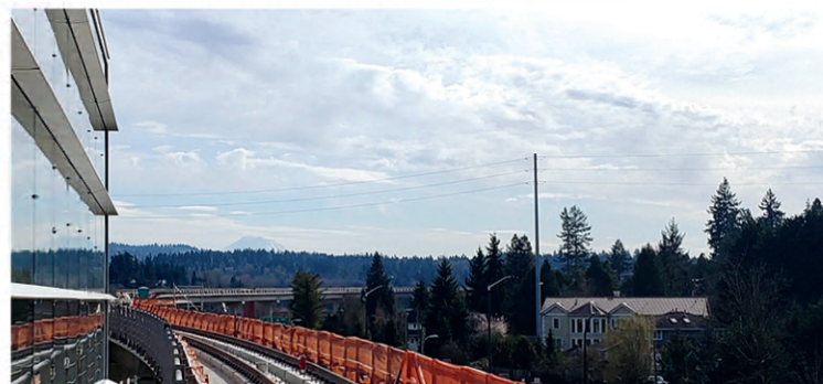
Atop the guideway at the South Bellevue light rail station (March 2020)
