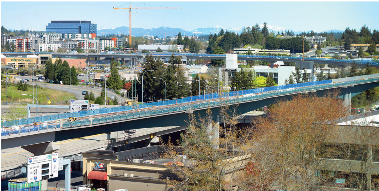
Current construction (April 2020)
