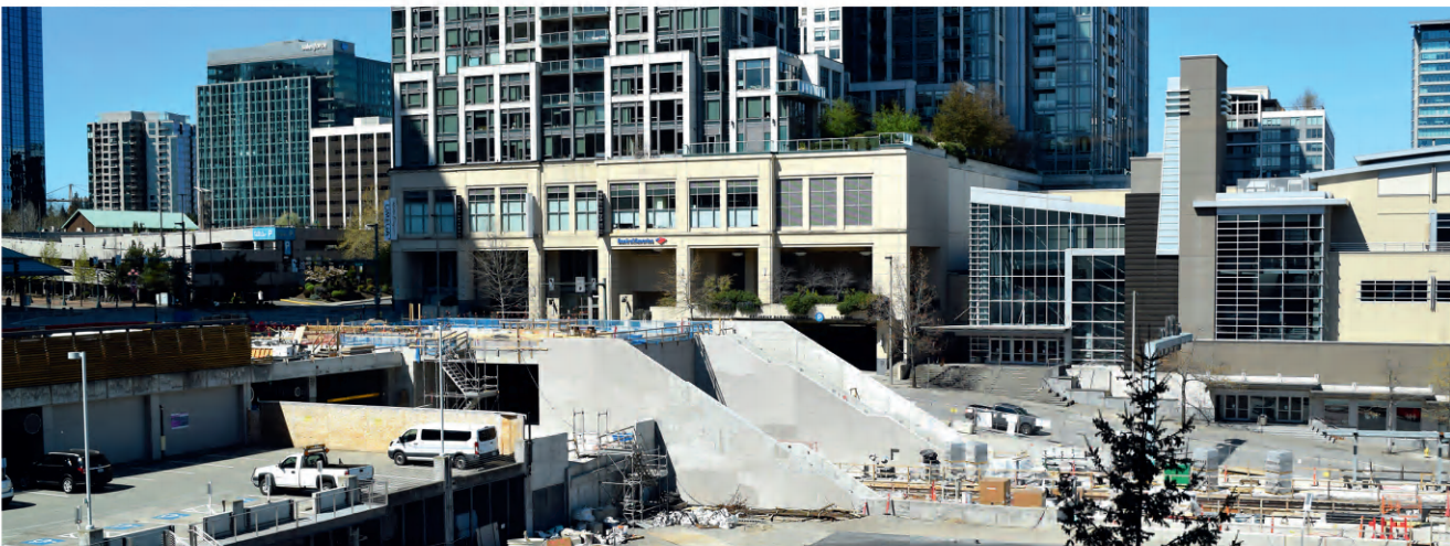
Current construction of Bellevue Downtown Station (April 2020)
