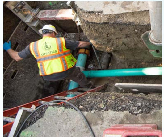
Replacement of Sewer Lines
