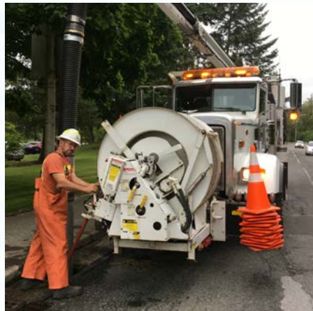
Vactor Truck Cleaning a Catch Basin
