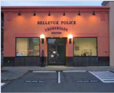
The Crossroads Community Station serves the surrounding residents and neighborhoods.
