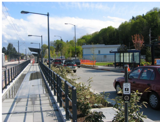
Figure 59 Bus stops in close proximity to light rail stations with short, direct pedestrian crossings make transit and pedestrian connections safe and convenient.
